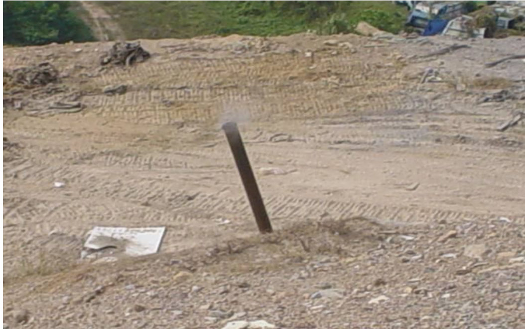
Plate 1.1: Passive release of landfill gas to the atmosphere (Fauziah, 2010).
