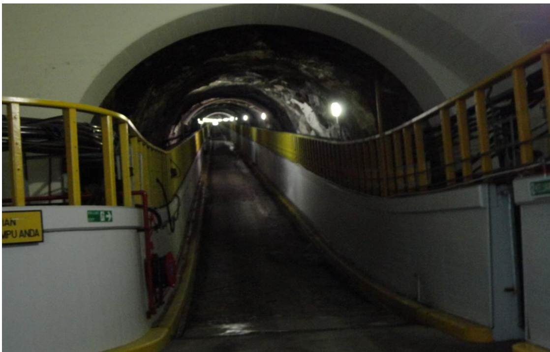
Jor underground power station hall access tunnel
