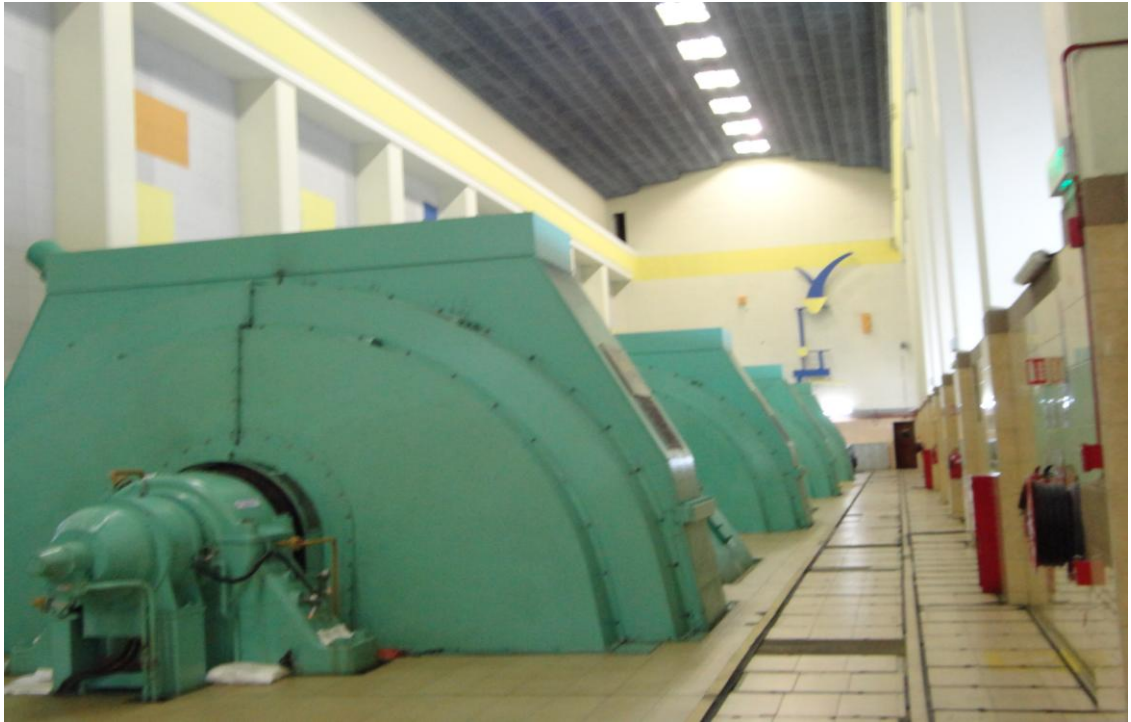
Jor underground power station hall
