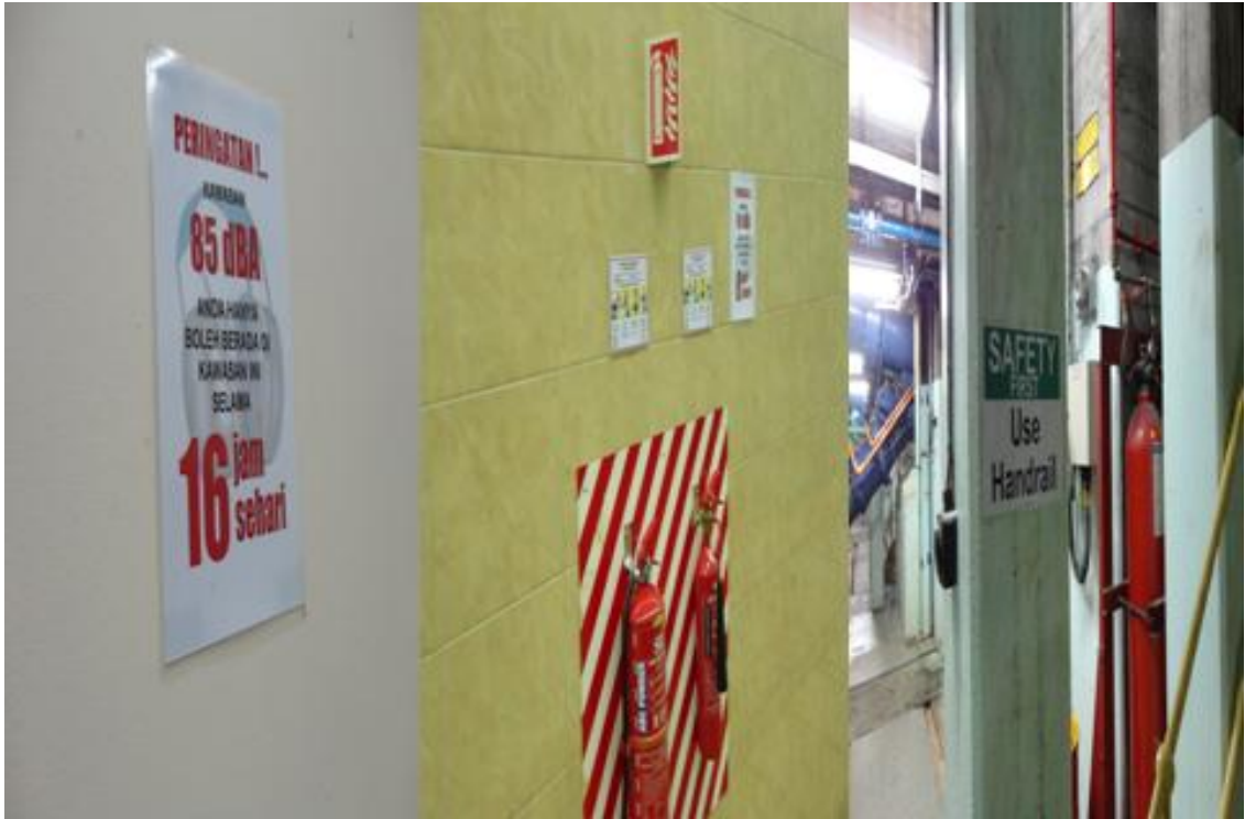
The symptoms of safety follow OSH regulation at JOR power station
