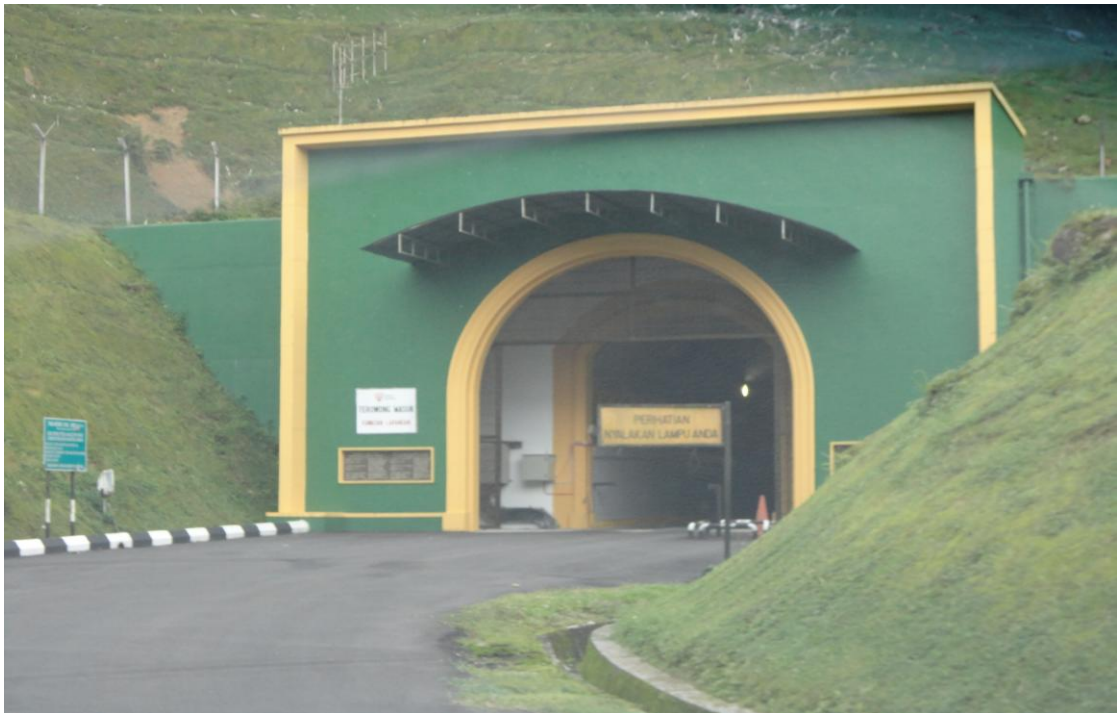
Jor underground power station hall entrance
