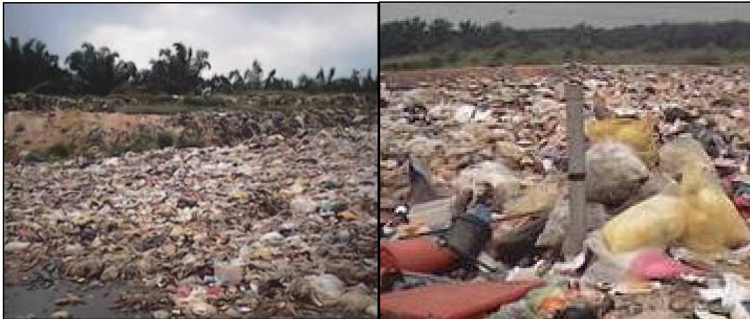
Plate 3.8: Waste cell and gas pipe at Ampar Tenang landfill.
