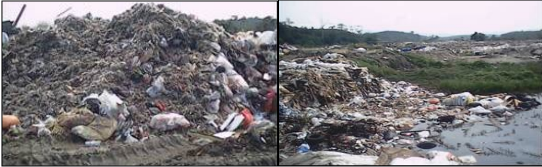
Plate 3.15: Active cells releasing leachate into the pond
