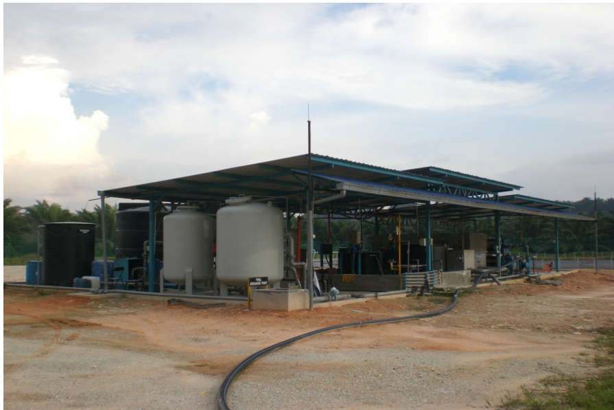
Plate 5.3: Leachate Treatment Plant
