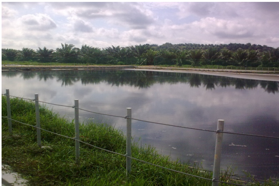
Plate 5.4 Leachate Retention Pond
