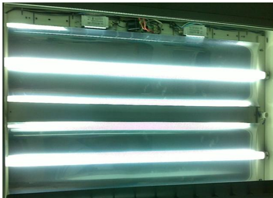
Figure 4.19: T8 lighting system in UM with ballast and starter
