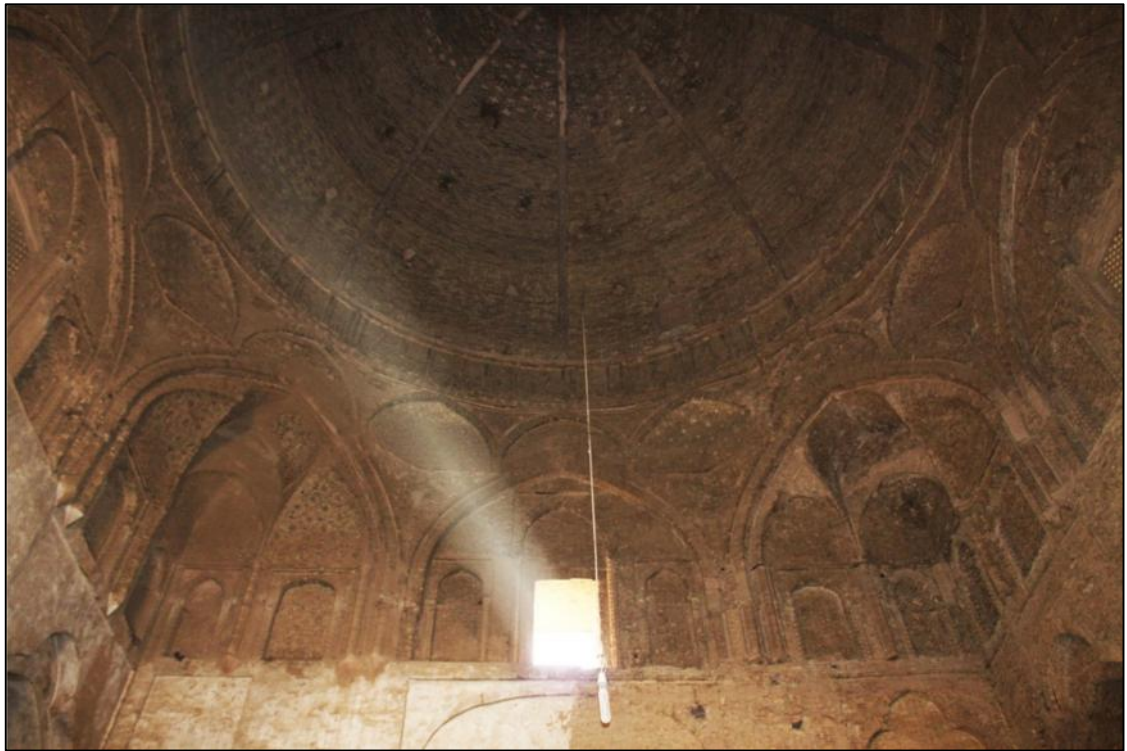
Figure 4.9 How the 4 sides of the square transformed into 8, 16 and then circle using arches. (Author)
