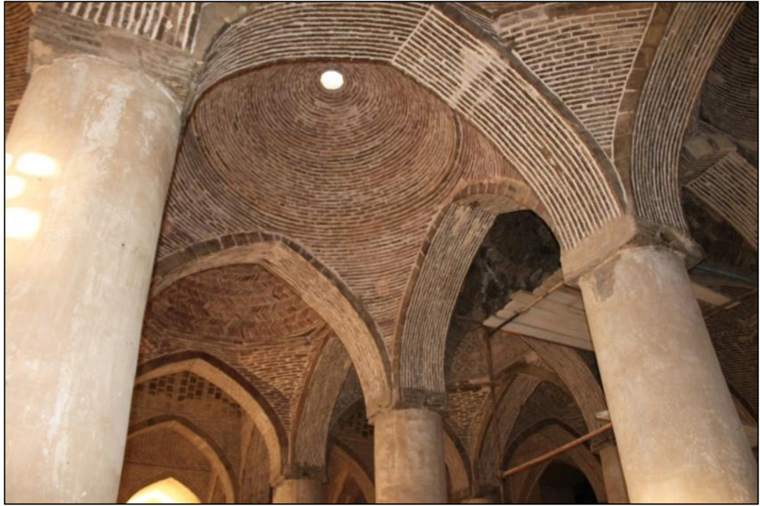
Figure 4.59 Structural arches mostly made in the pointed format. (Author)
