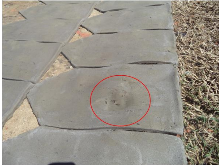
Figure 4.29: Unevenness on the surface of green tiles Source: Field study (2013)
