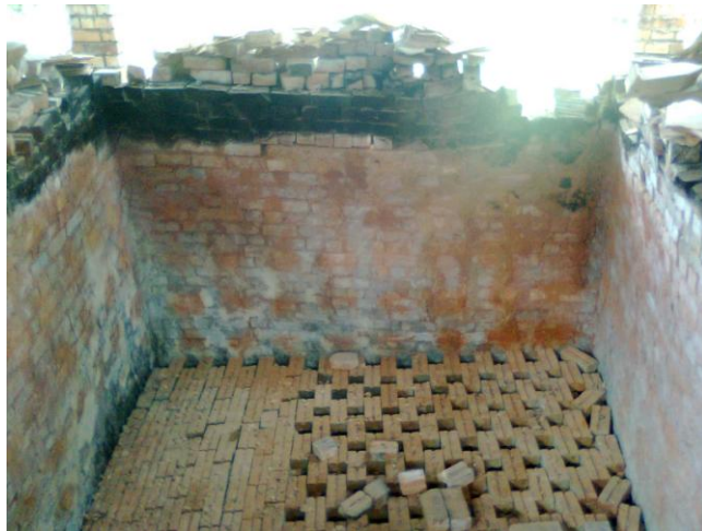
Figure 4.19: The arrangement of bricks in the base of kiln's chamber Source: Field study (2013)
