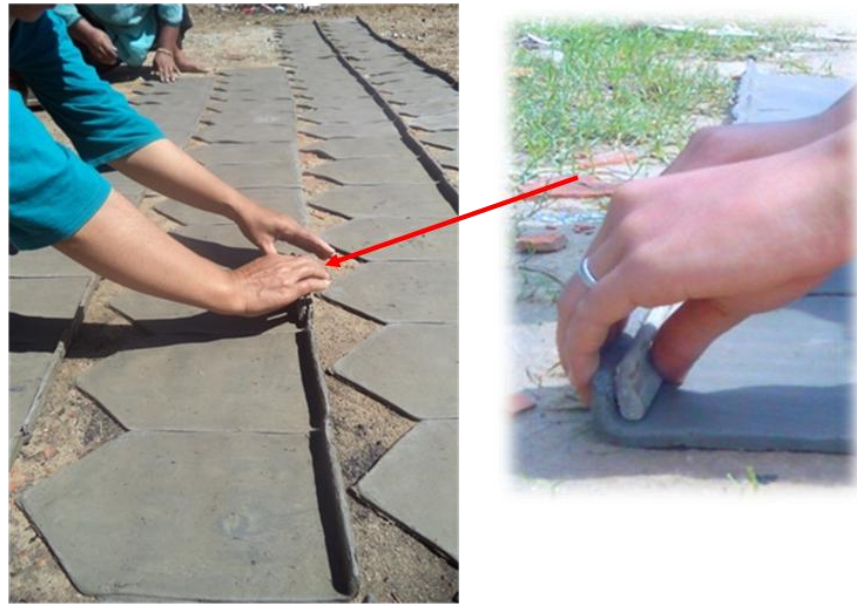
Figure 4.8: The end area of body tile was bent upright to form the hook Source: Field study (2013)
