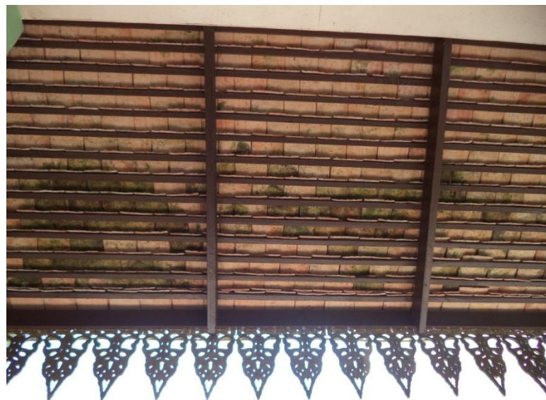
Figure 1.5: The installation of Singgora tiles on the battens Source: Field study (2013)
