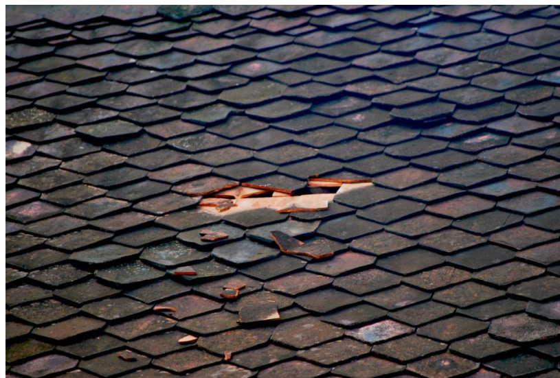
Figure 1.3: Broken Singgora tiles on the roof Source: Field study (2013)
