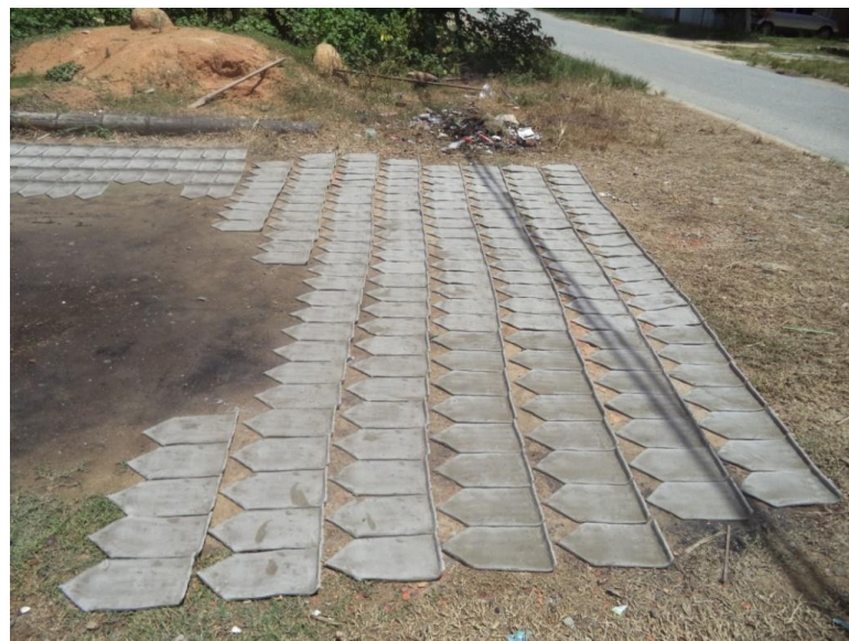
Figure 4.7: The tiles were dried naturally outdoors and laid on the ground Source: Field study (2013)
