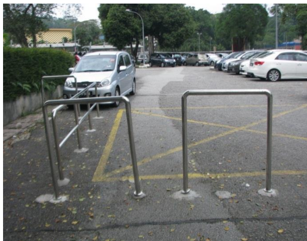
Figure 5.14: Architectural barrier at the end of the car park
