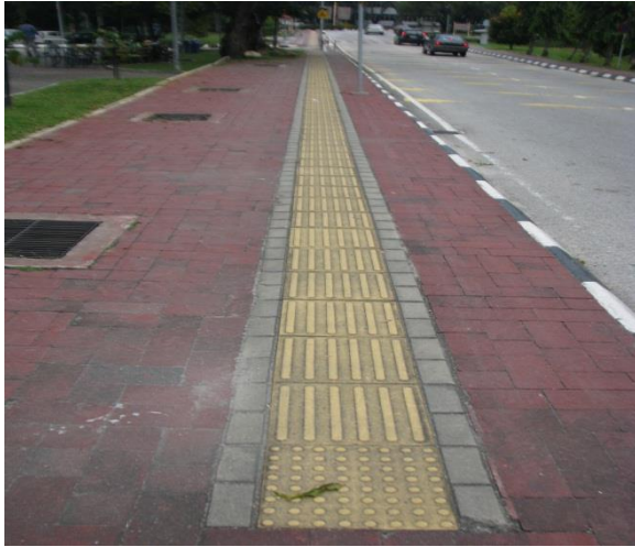
Figure 5.26: Tactile paving in front of library
