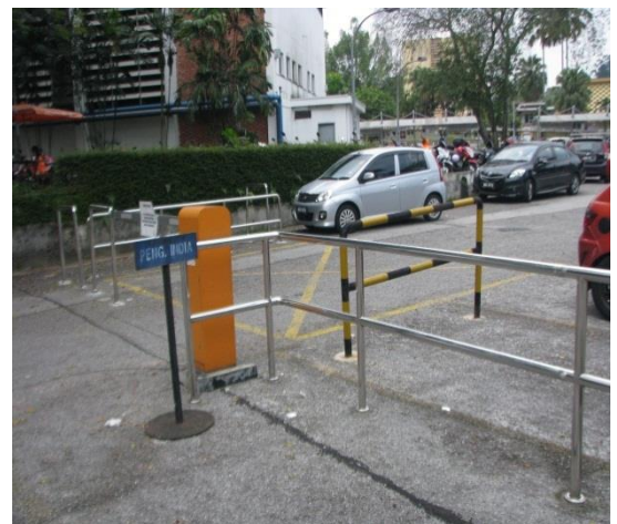
Figure 5.15: Architectural barrier at the end of the car park
