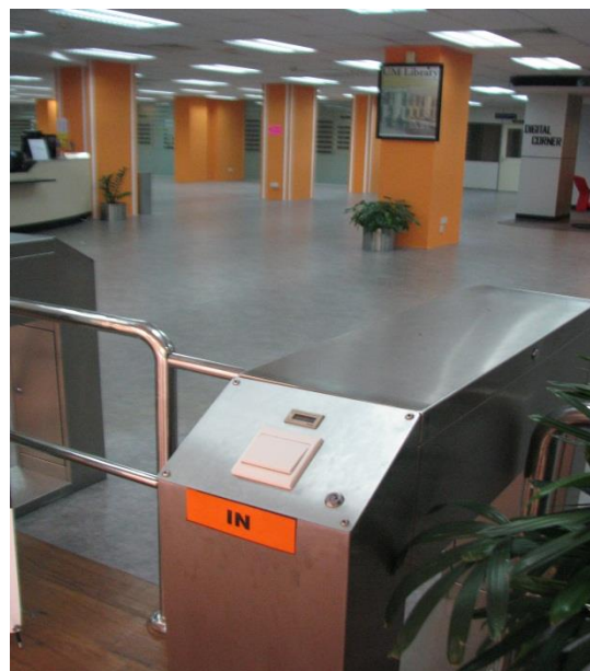
Figure 5.31: Lack of Tactile path inside library
