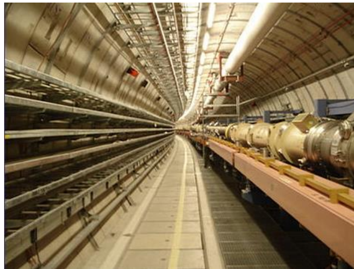
Figure 3.5: A small segment of the HERA tunnel. The proton beam is travelling in the large vacuum tube in the middle to the right while the electron beam tube is below that.
