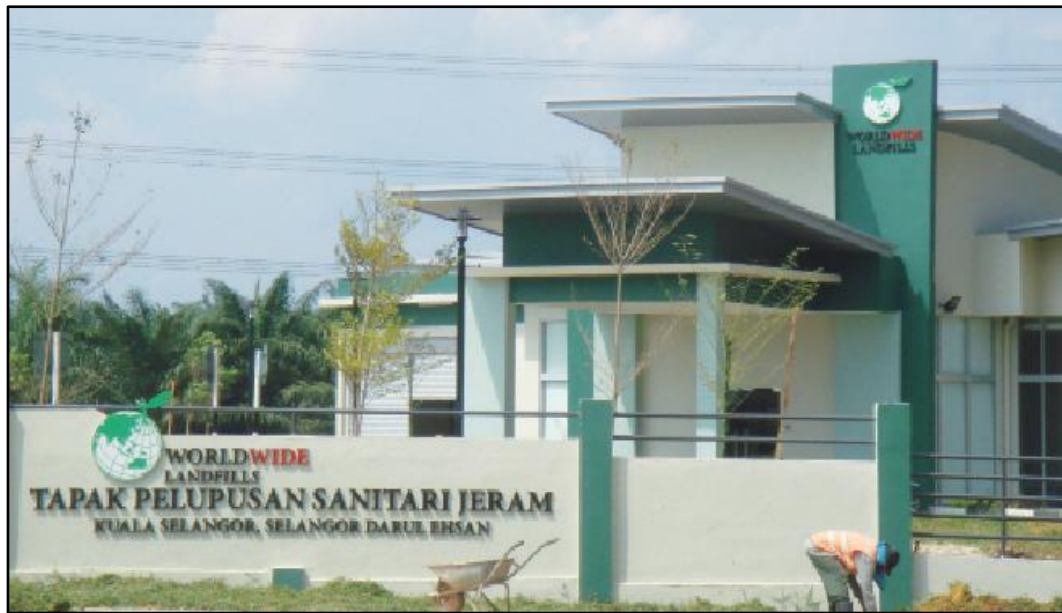
Plate 3.1: Jeram Sanitary Landfill entrance
