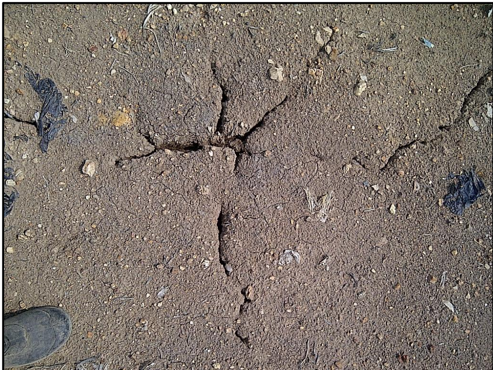
Plate 4.2: Visible cracks on JSL cover soil during dry period
