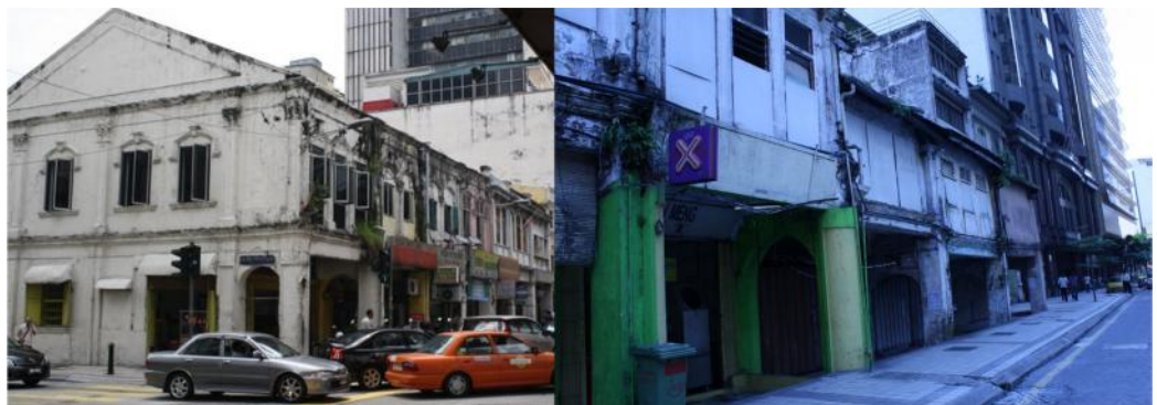
Old ruined buildings and dirty facades in Tun Perak Street
