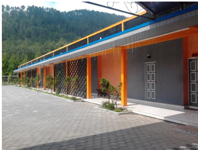
Figure 4. Karaoke and operator's room, South Part
