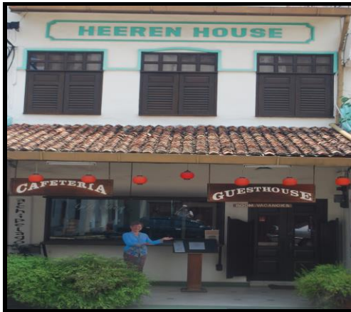
Figure 7.12: Two Former Warehouses/ Heeren -house. Jalan Tun Tan Cheng Lock, Melaka.
