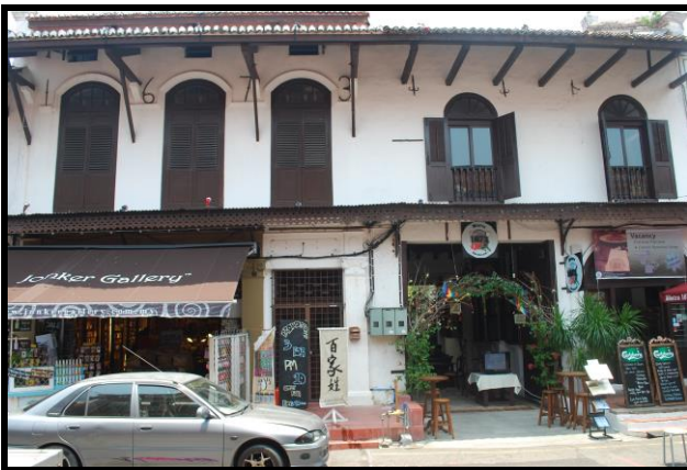
Figure 7.13: VOC Building (1673). Jalan Hang Jebat, Melaka. Source: R.C.M. Weebers.
