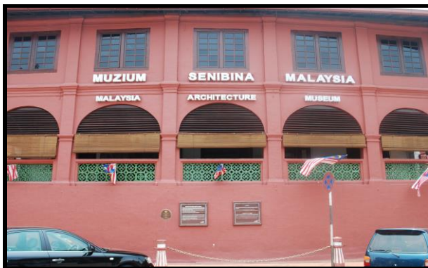
Figure 7.7: Architecture Museum (18 th century). Jalan Kota, Melaka. Source: R.C.M. Weebers.
