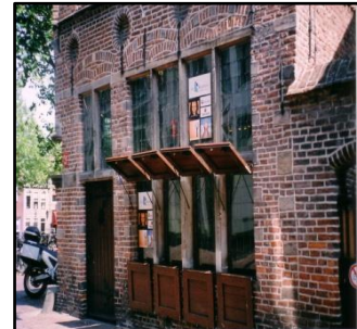
Figure 8.7: Krankeledestraat 111. Amersfoort, the Netherlands. Source: R.C.M. Weebers
