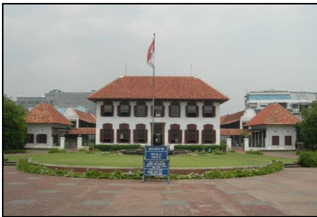
Figure 5.19: Jakarta/Batavia, Java. The Reynier de Klerk House (1760). Source: http://www.panoramio.com .
