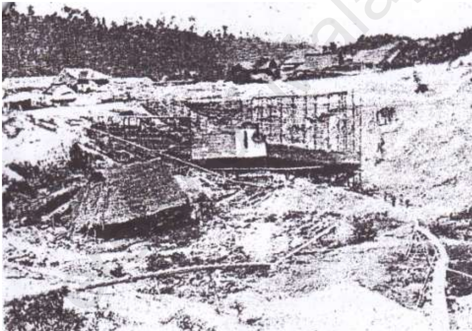
Figure 5.14: One of the mines found in Sungai Raia
