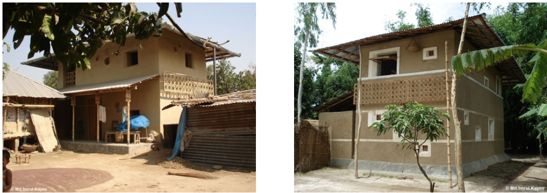
Figure 2.3: Local earthen construction practice was improved to protect against rain and rising damp. The external walls are left while internal walls are plastered with clay plaster with light-coloured white mud.
