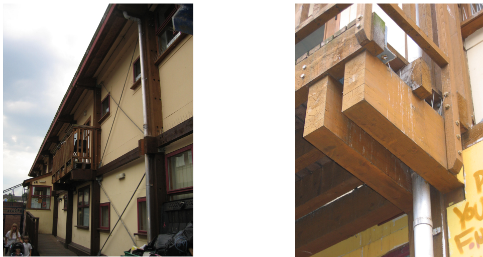
Figure 2.5: Community Centre at St. Annes, Nottingham departed from Segal's approach. Construction at the balcony using bolts and nuts.
