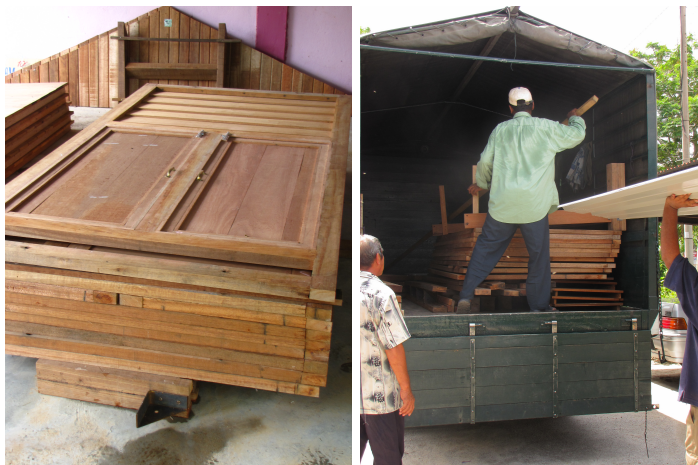
Figure 5.35: Stacking the Panels as Means of Storing and Delivering
