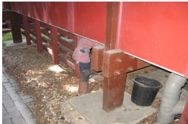
Figure 5.6: Pad Foundation Used for Self Build Housing at Segal Close Source: Author's collection
