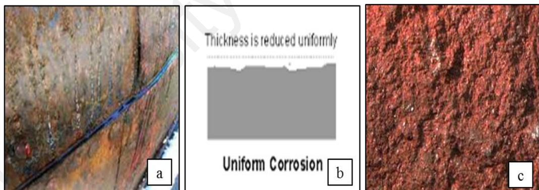
**Figure 2.5:** Uniform Corrosion
