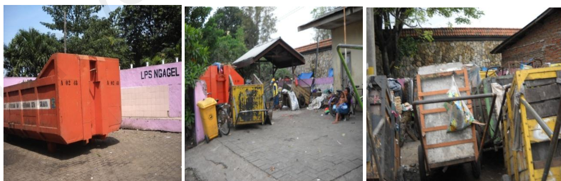
Figure 4.3. Current Condition of Several Waste Transfer Stations in Surabaya (Personal Documents, Fieldwork, December 2010)
