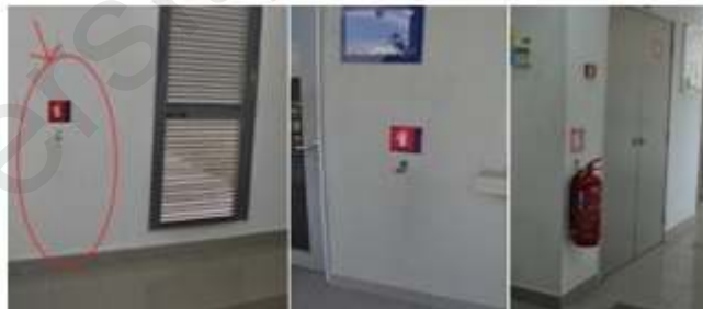
Fire prevention services - fire fighting system is functioning but some of the fire extinguishers were not found during the survey
