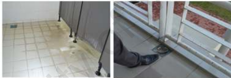
Plumbing services – leakage of fittings, the cover of floor traps were not properly closed
