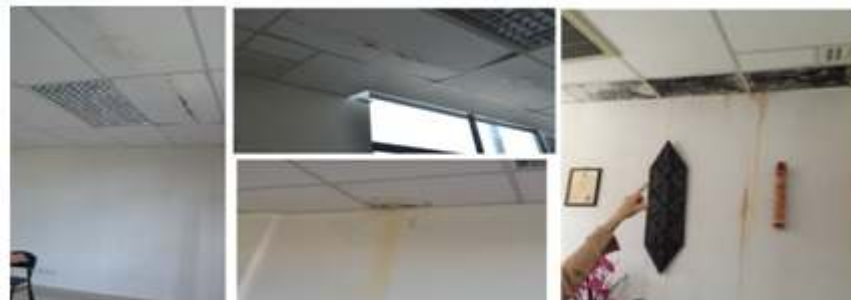
Roof and ceiling finishes - leakage at the ceiling of several lecture halls, classrooms and lecturers' room due to poor waterproofing of roof
