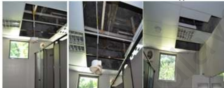
Electrical services - Improper installation of electrical wiring were found in the toilet (ground floor level)
