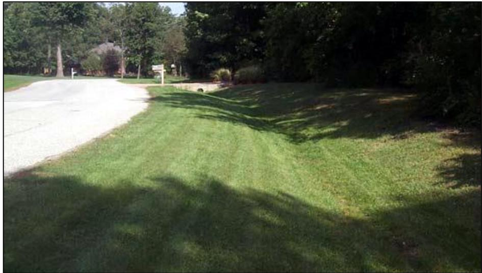
Figure 2.13: Constructed grass swale
