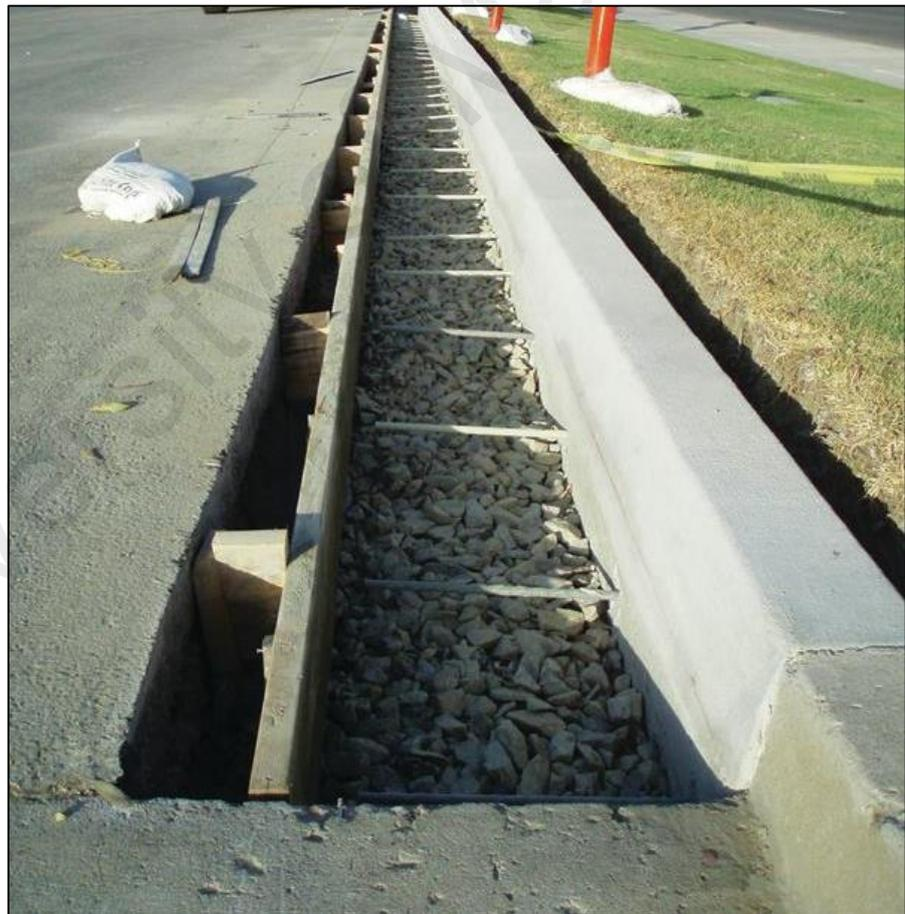
Figure 2.12: Infiltration trench constructed in highway
