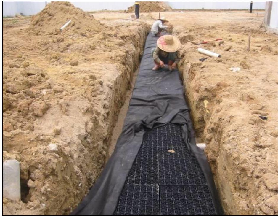
Figure 2.17: Constructed Modular system as conveyance system
