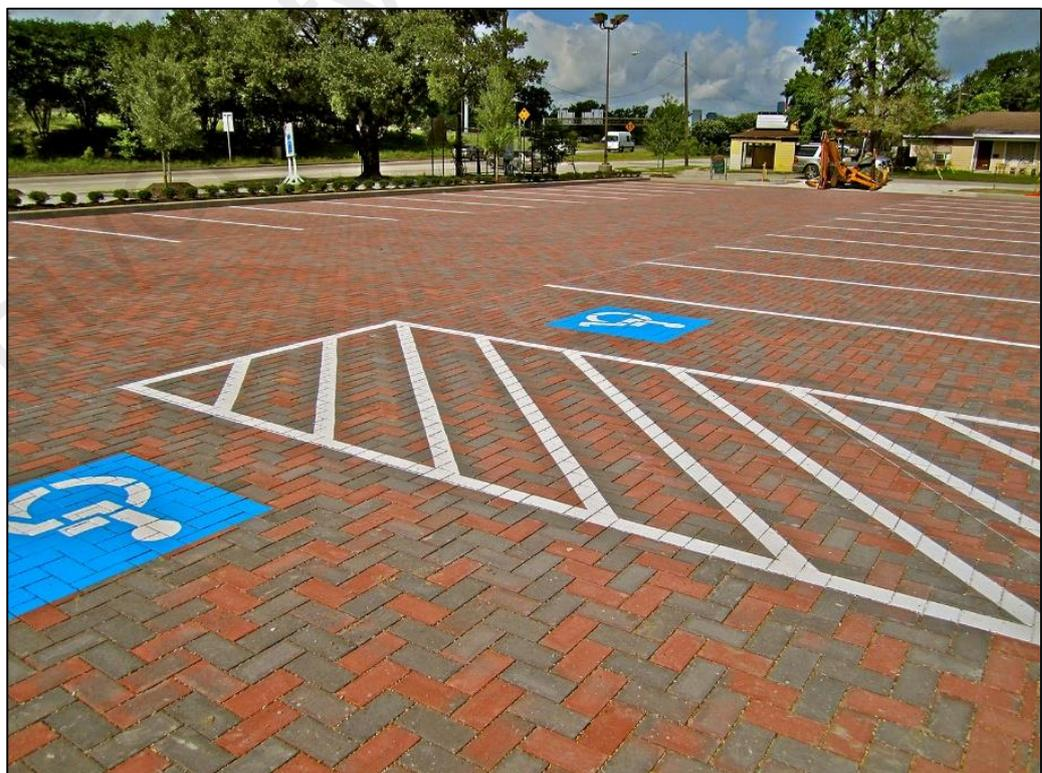
Figure 2.6: Pervious surface constructed in the parking lot
