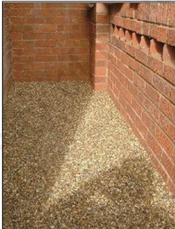
Figure 2.7: Gravelled area to increase the infiltration of surface
