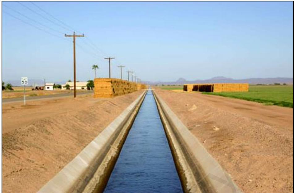
Figure 2.14: Concrete channel constructed to transfer the water
