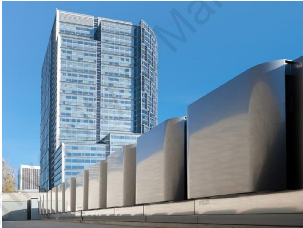
Figure 2.9: Fuel cells used for building (source: http://www.fuelcells.org/uploads/bloom_constellation-place.jpg )
