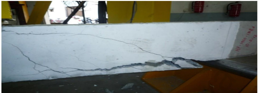
Figure 4.21: Debonding failure mode of H1B8F19L80W1.2T
