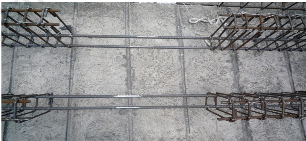
Figure 3.8: Surface preparation of steel bars to place strain gauges
