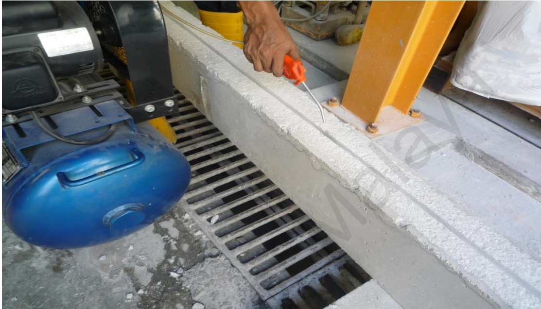
Figure 3.4: Compressed air jetting
