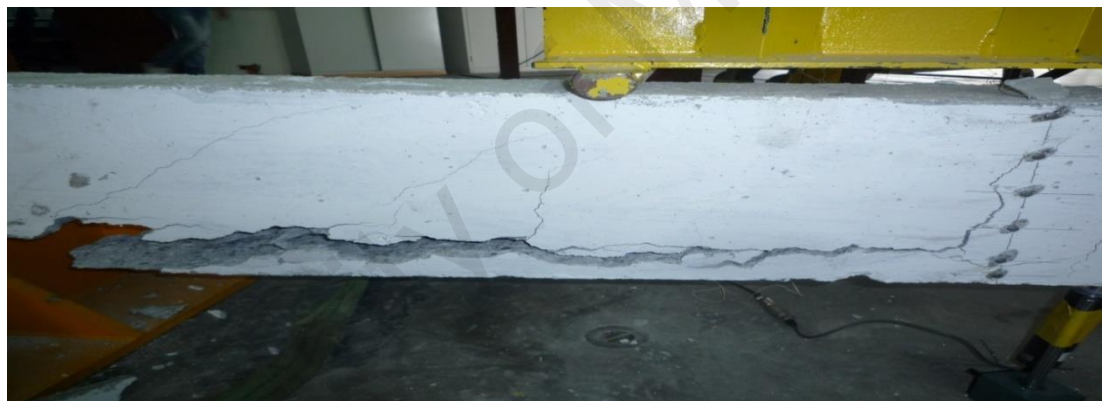
Figure 4.22: Debonding failure mode of H1B8F16L80W1.2T
