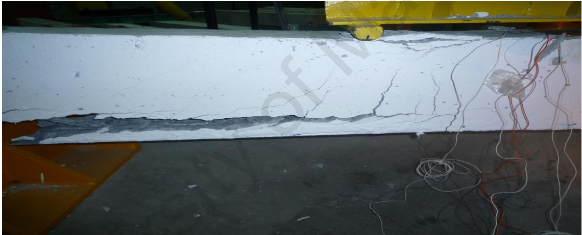
Figure 4.7: Debonding failure mode of H2B6S19L125W2T
