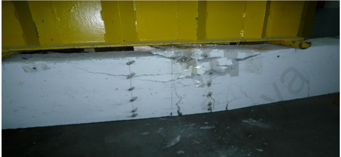
Figure 4.36: Failure mode of control beam
