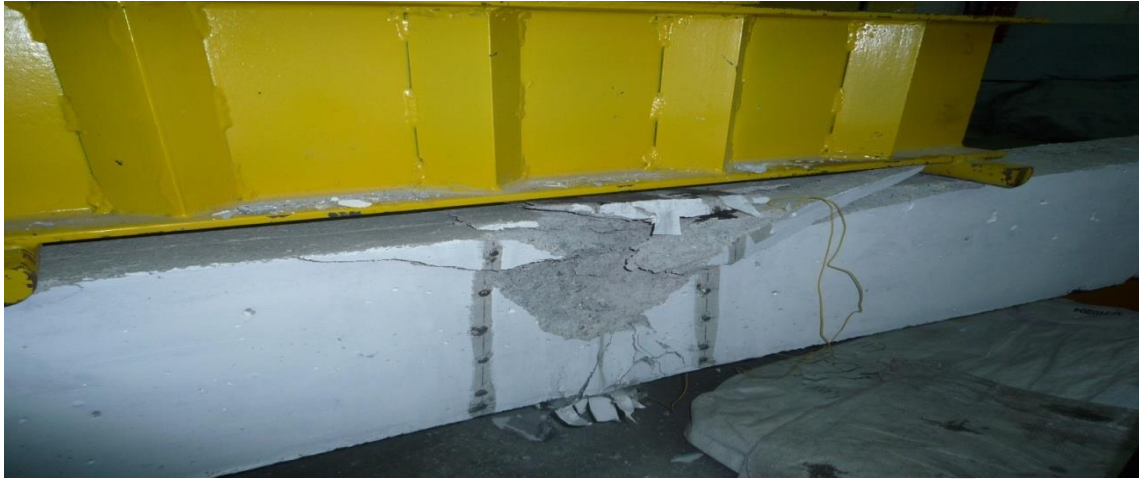
Figure 4.27: Flexure failure mode of H1B6FR19L100W.17T
