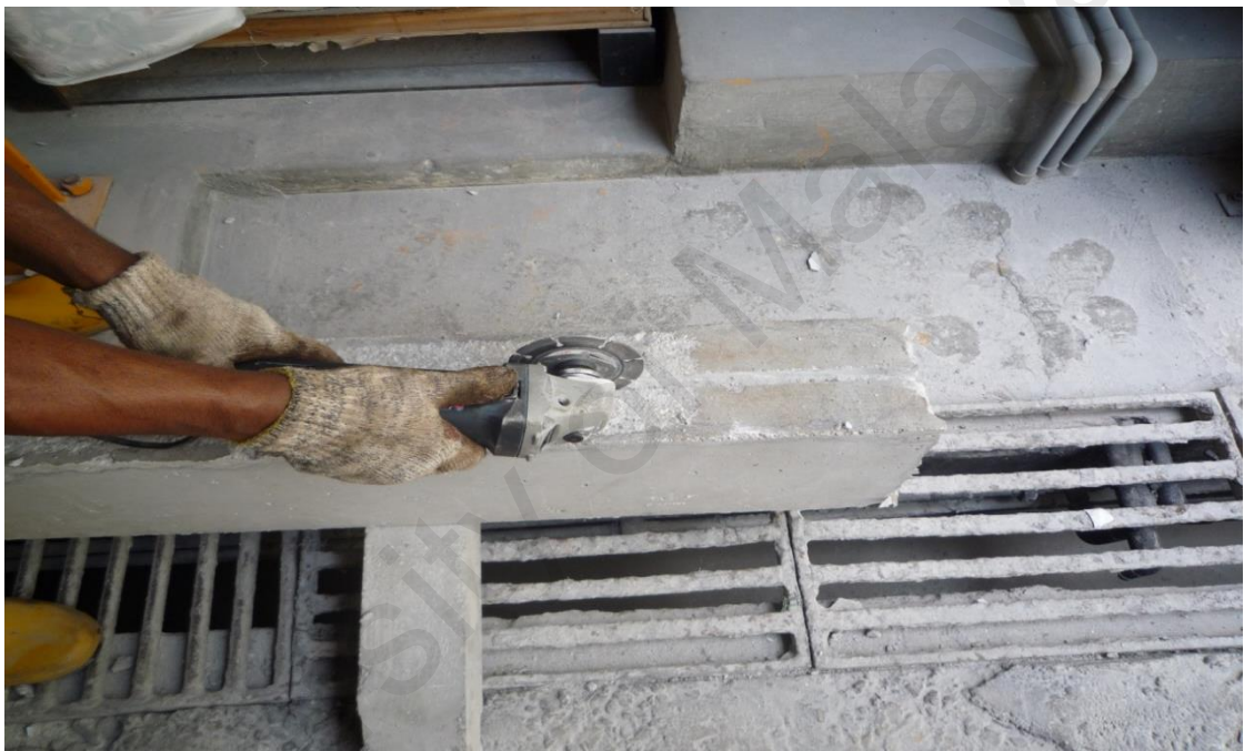
Figure 3.6: Groove cutting
