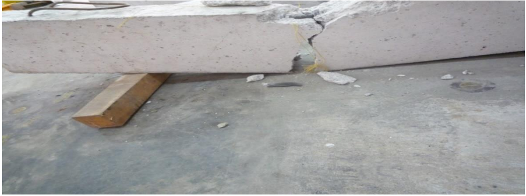
Figure 4.56: Fatigue failure mode of control beam
