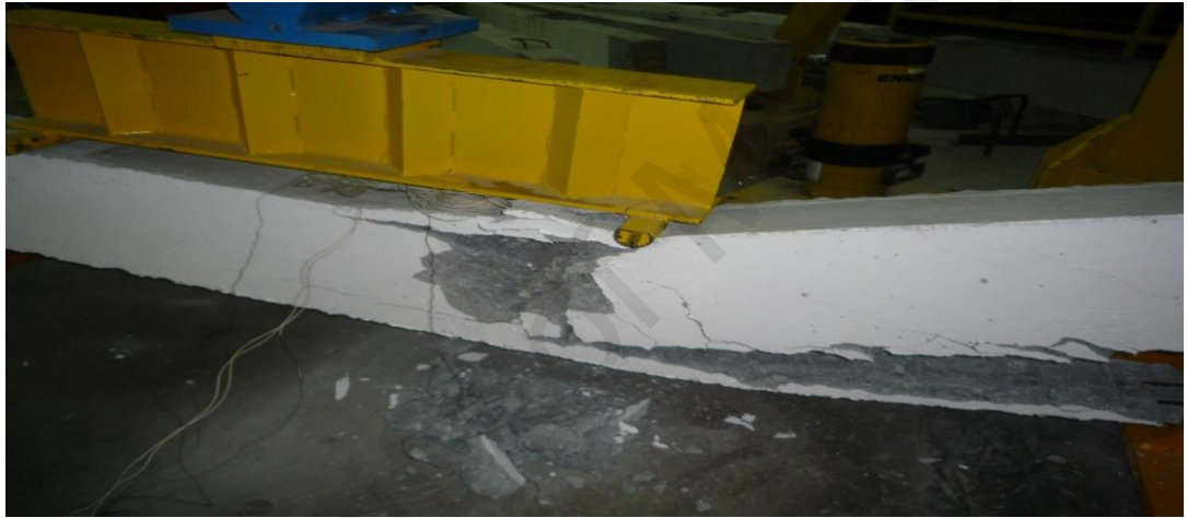
Figure 4.4: Debonding failure mode of H2B8S19L73W2T
