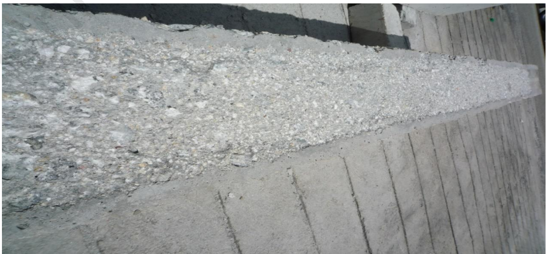
Figure 3.3: Prepared surface of a concrete beam
