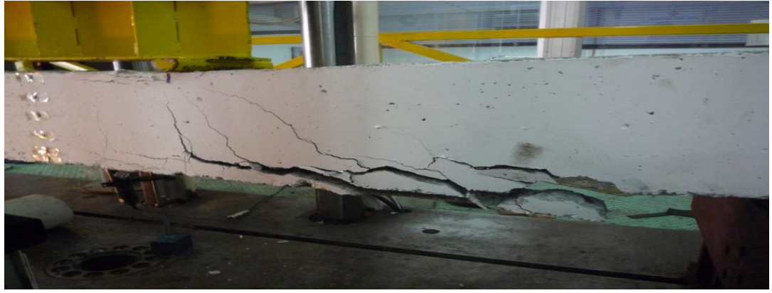
Figure 4.3: Debonding failure mode of H1B6S16L73W2T
