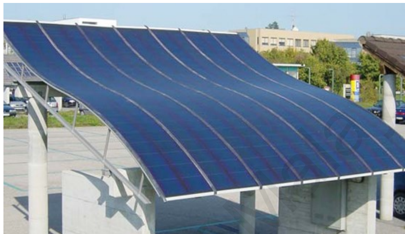
Figure 2.14: Amorphous PV panel on a garage roof (Renewables, 2010)
