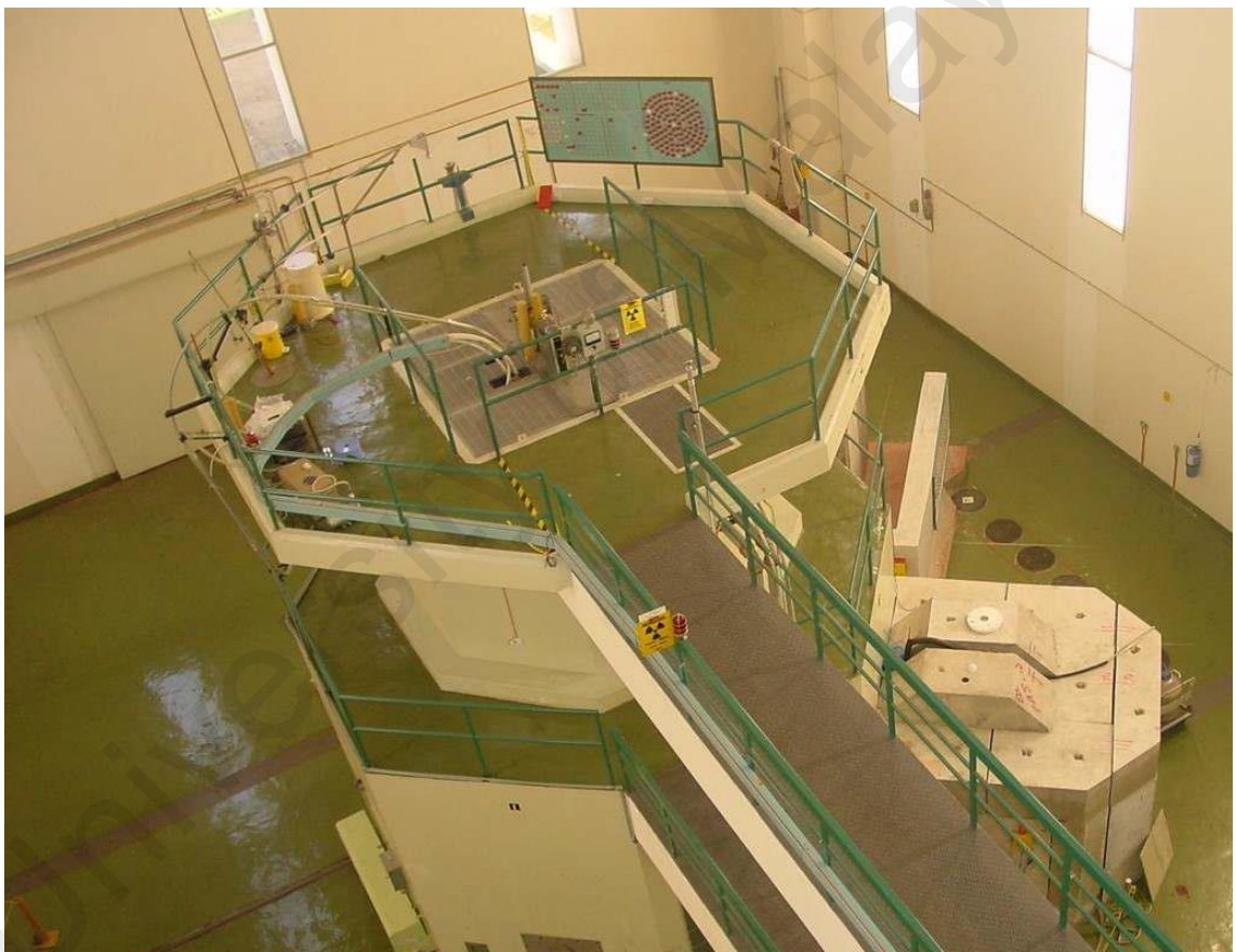
Figure 3.4: The top view of the TRIGA PUSPATI Reactor in Malaysia Nuclear Agency, Bangi (Mohamed Takip, 2009), which is a 7 m high pool type reactor surrounded by high density concrete.
