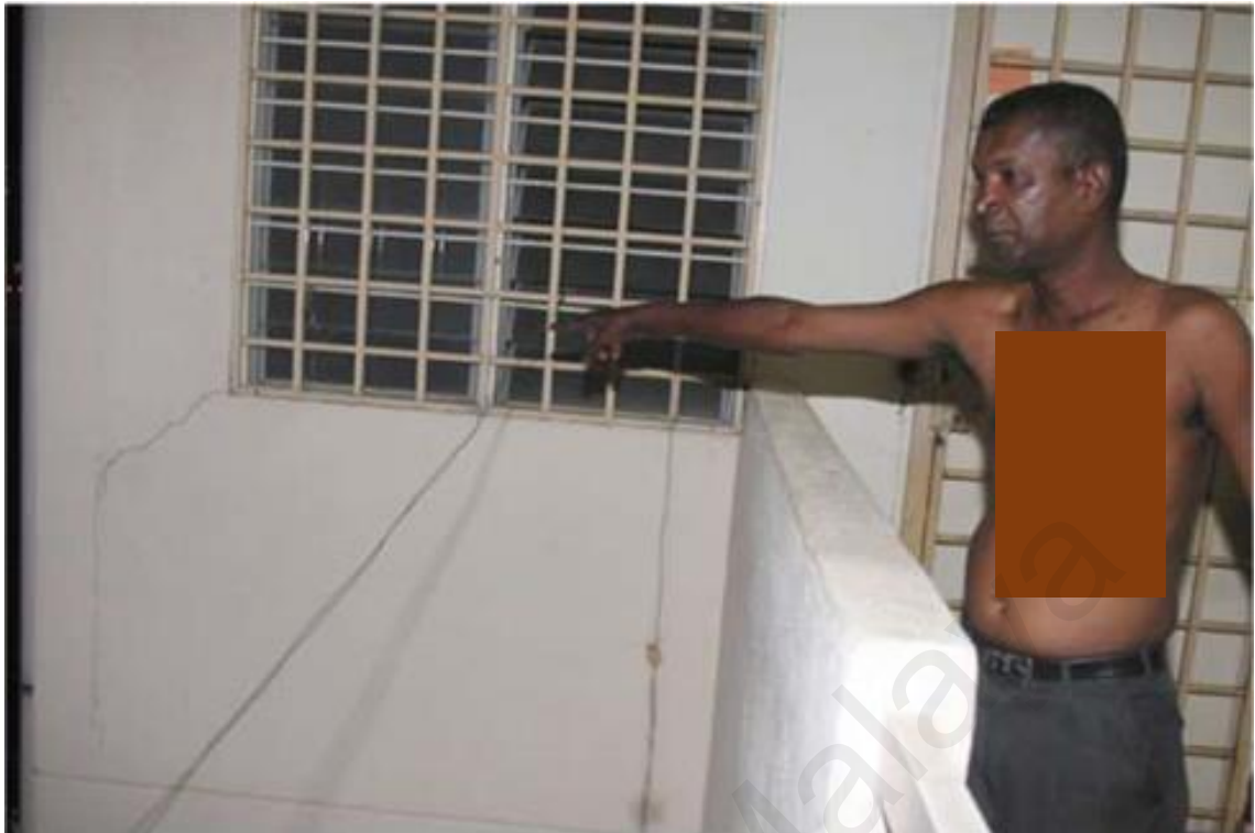
Figure 1.4: Observed damage to the Pantai Dalam flats after the southern Sumatra earthquake, Sept. 30, 2009.
