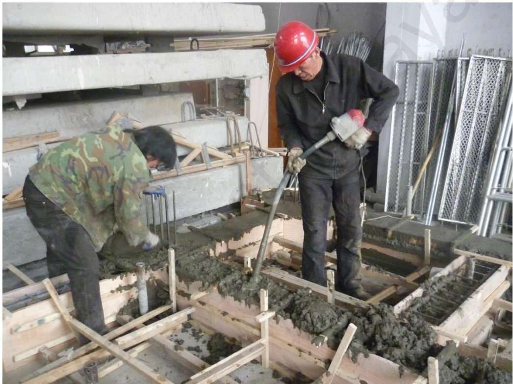
Figure 4.11: Construction of RC based beam.
