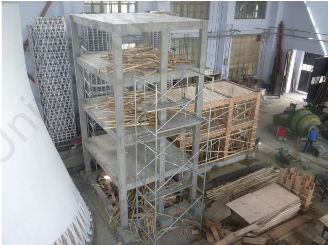
Figure 4.17: The scaled model after stripping forms.
