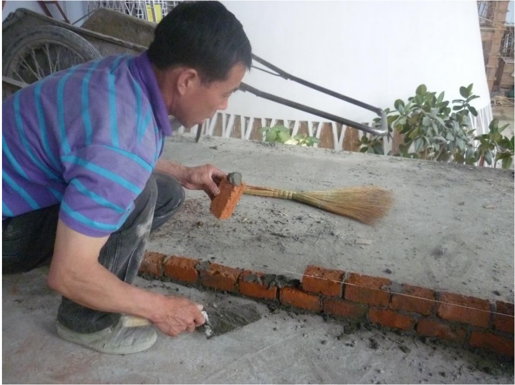
Figure 4.20: Construction of unreinforced masonry infill walls.
