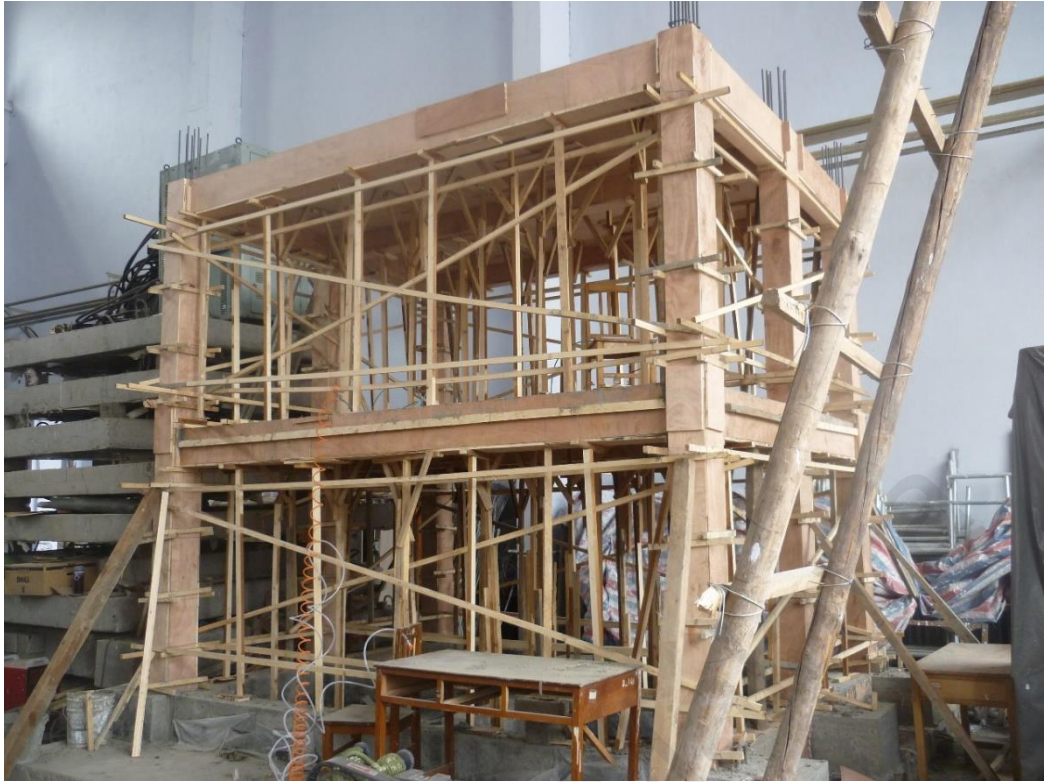
Figure 4.12: Formwork for the scaled model.
