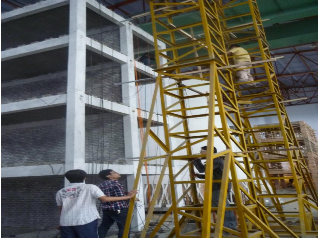
Figure 4.8: Installation of LVDTs.
