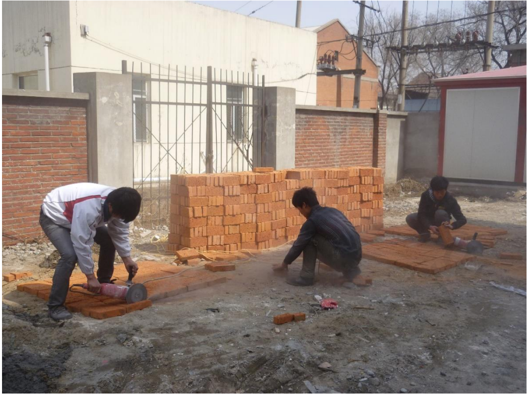
Figure 4.18: Cutting solid clay bricks.
