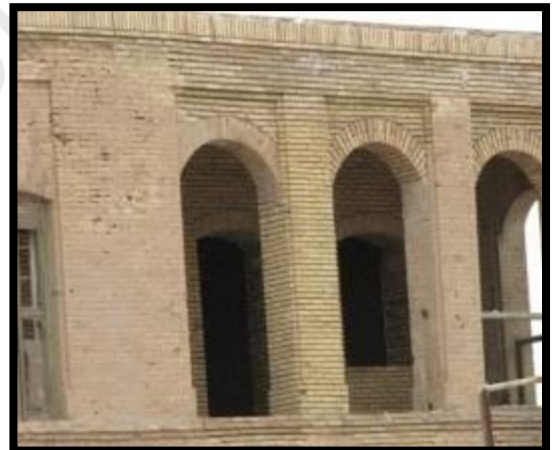
Figure 5. 3: Brick used in pre-war buildings of Khorramshahr
