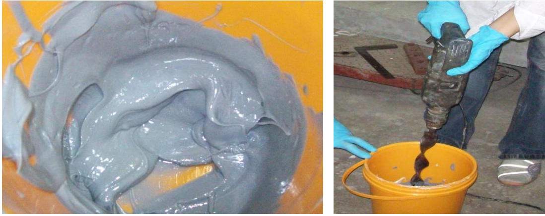
Figure 3.6 Mixing of components A and B (Sikadur®-330)
