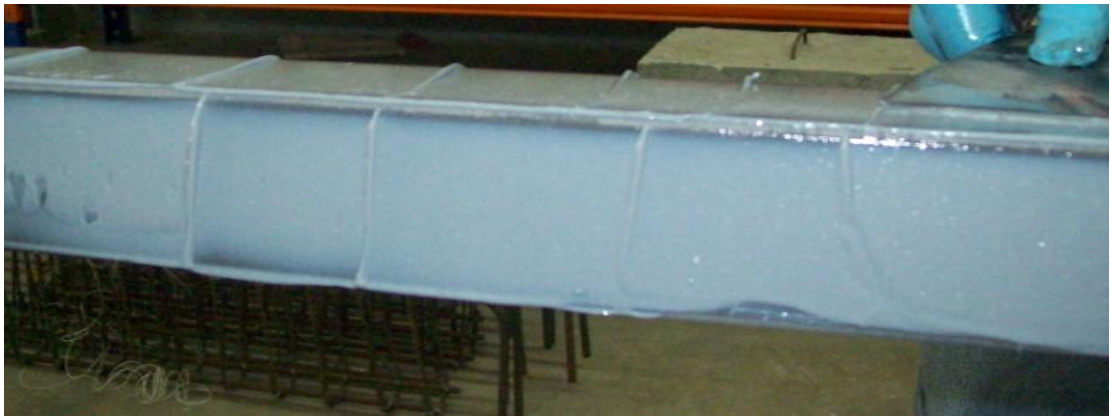
Figure 3.7 Applying epoxy onto the surface of the SHS
