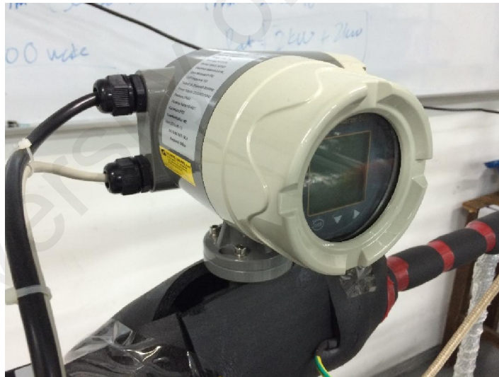
Figure 3.9 Photograph of the Electromagnetic flow meter
