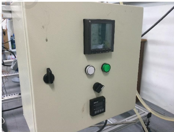
Figure 3.19 Photograph of the heating control units
