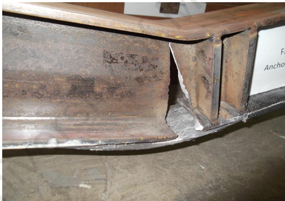
Figure 4.47: Failure mode of anchored specimen with CFRP fabrics (F7) under fatigue
