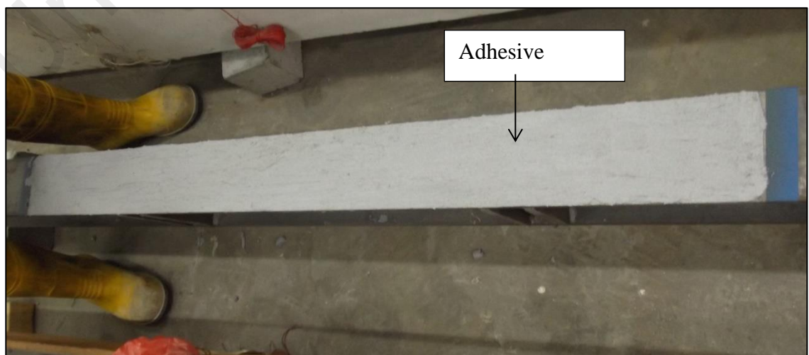
Figure 3.19: Applying adhesive on the surface of the beam flange
