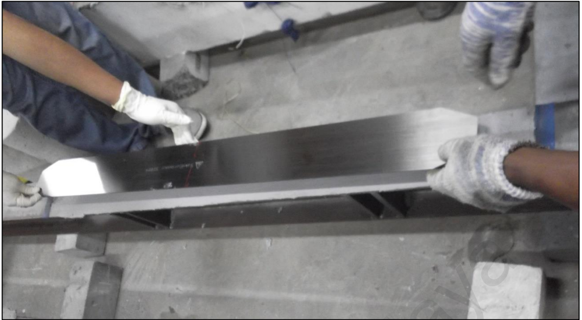
Figure 3.20: Placing of the CFRP plate
