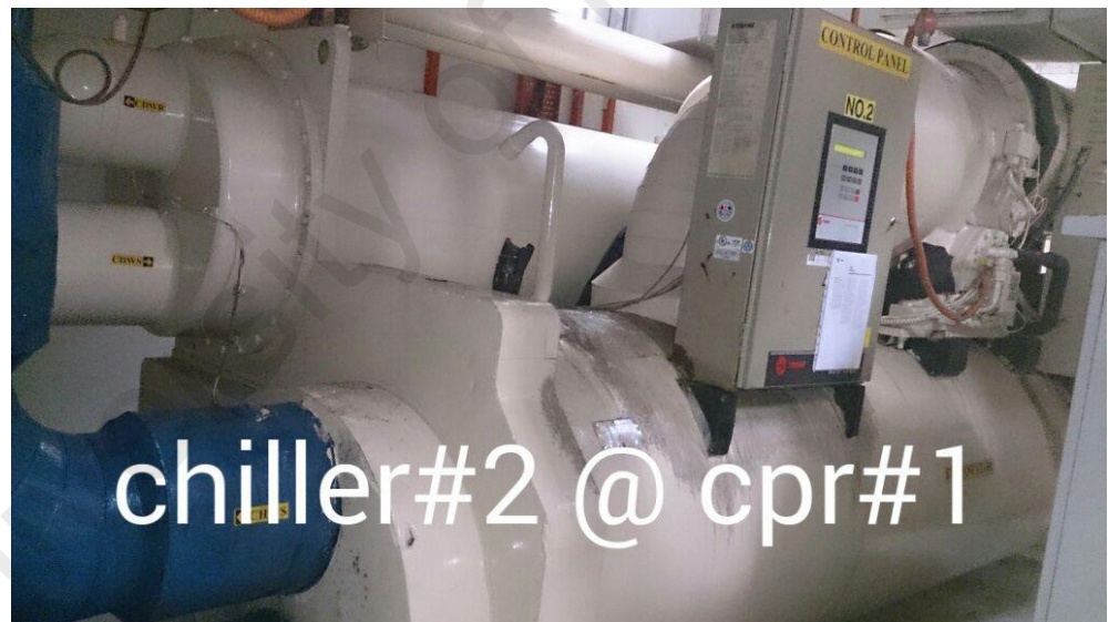
Figure 3.2 - Existing Carrier Chiller Number Two at the CPR-1.
