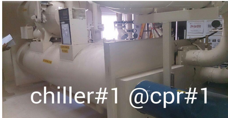
Figure 3.1 - Existing Trane Chiller Number One at the CPR-1.
