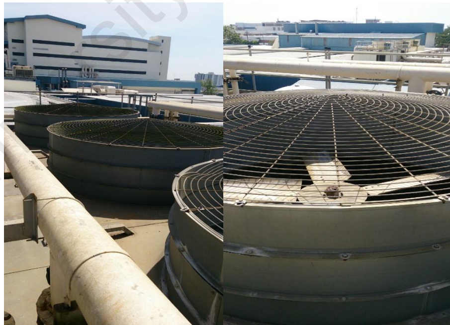
Figure 3.6 - Top view for the Existing Cooling Towers for the CPR-1.
