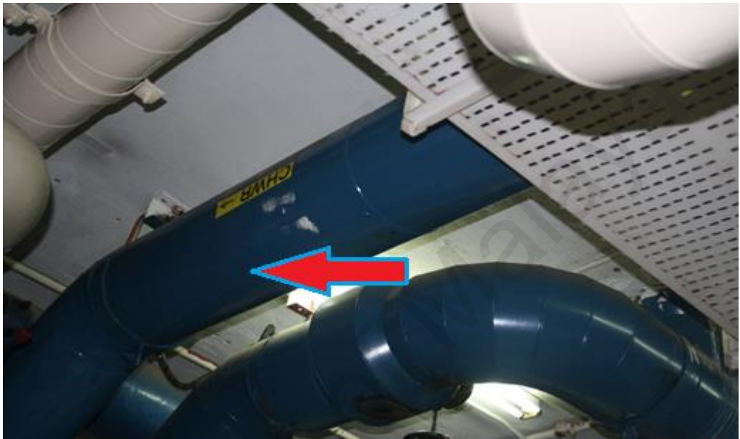
Figure 3.13 – Ultrasonic flow location for chilled water Supply line at Chiller 1
