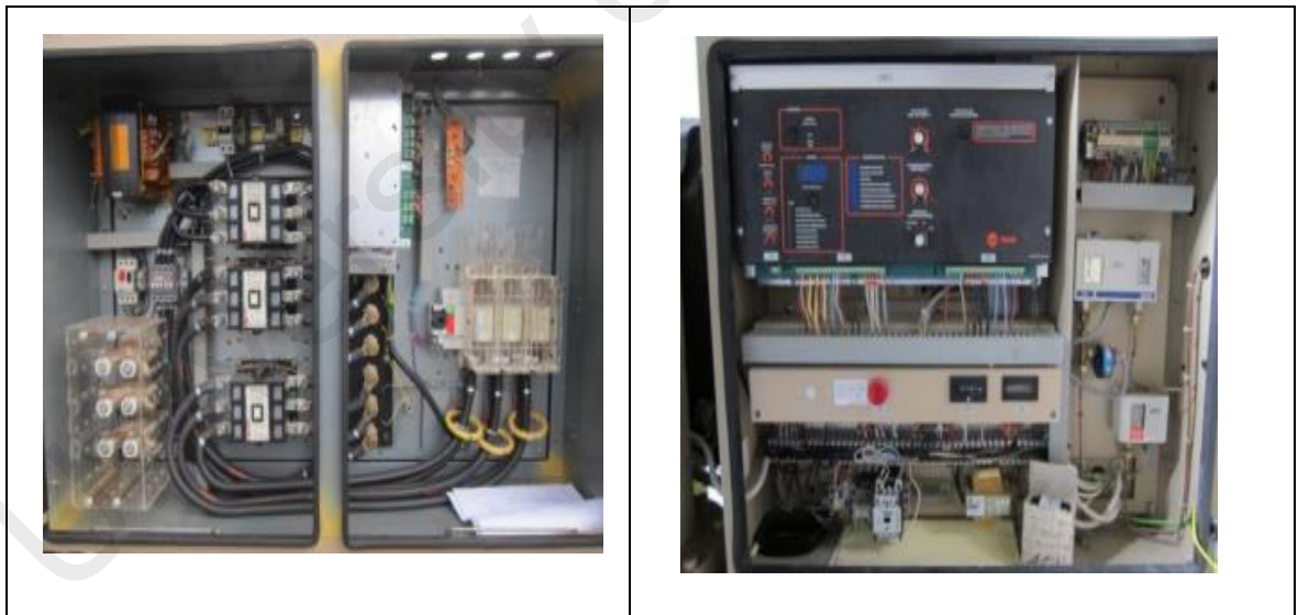
Figure 2.12: Electrical Control Panel (Noria , 2015)
