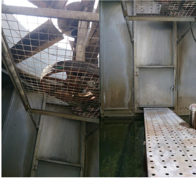
Figure 3.7 - Interior look for the Existing Cooling Towers for the CPR-1.
