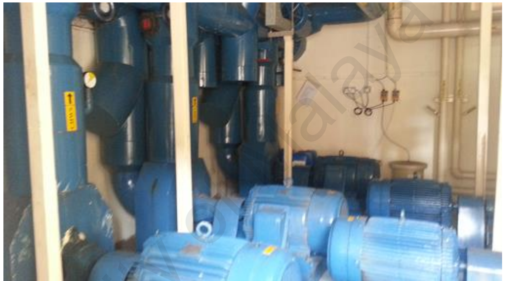
Figure 3.3 - Existing Chilled Water Pumps at the CPR-1
