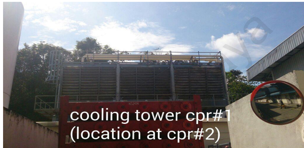
Figure 3.5 - Existing Cooling Towers for the CPR-1
