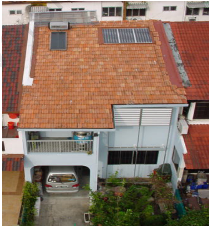
Figure 2.7: CETDEM Demonstration house in Petaling Jaya (CETDEM, 2011a)
