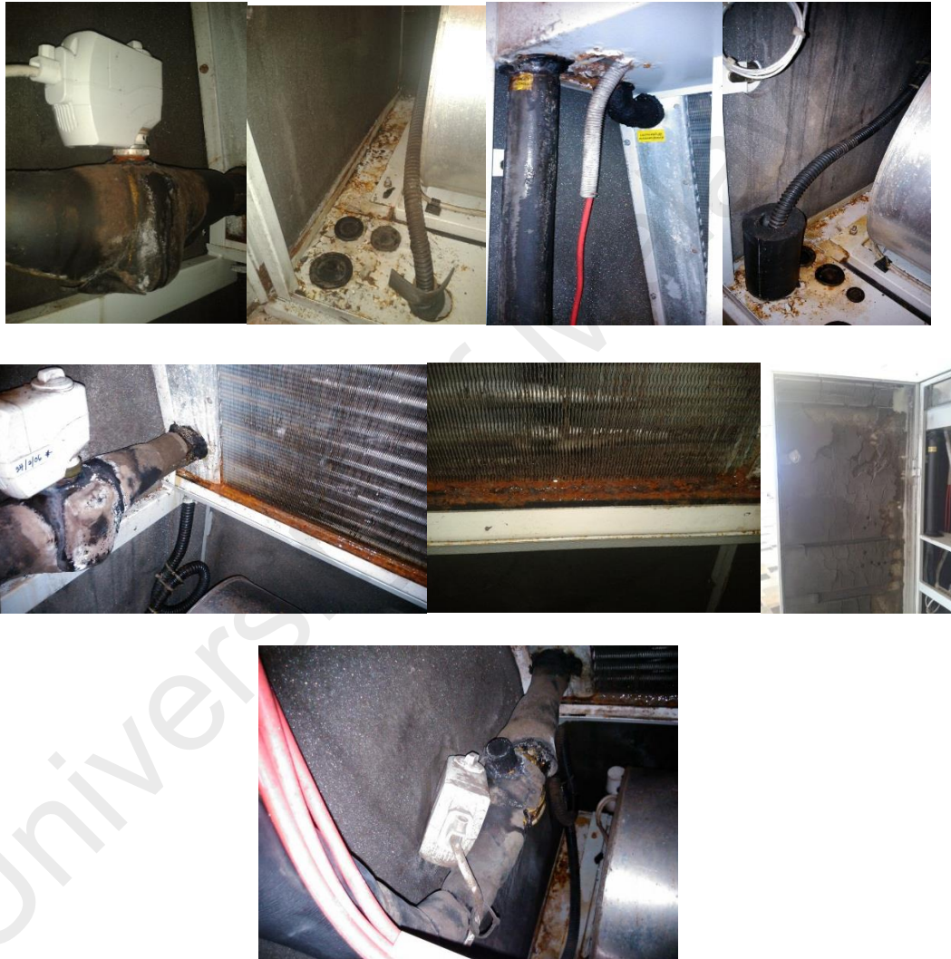
Figure 4.14: The internal conditions of the AHU units.
