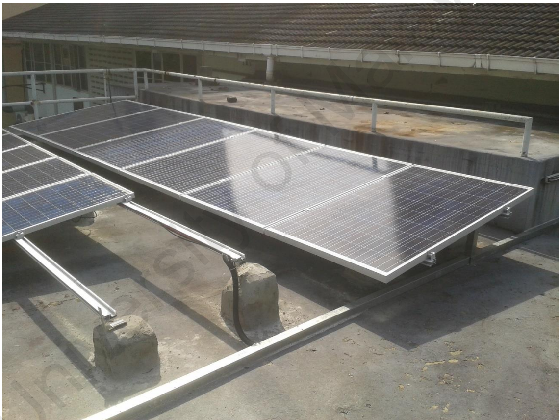
Figure 3.4: Experimental setup of the 1 kW on-grid solar photovoltaic system.
