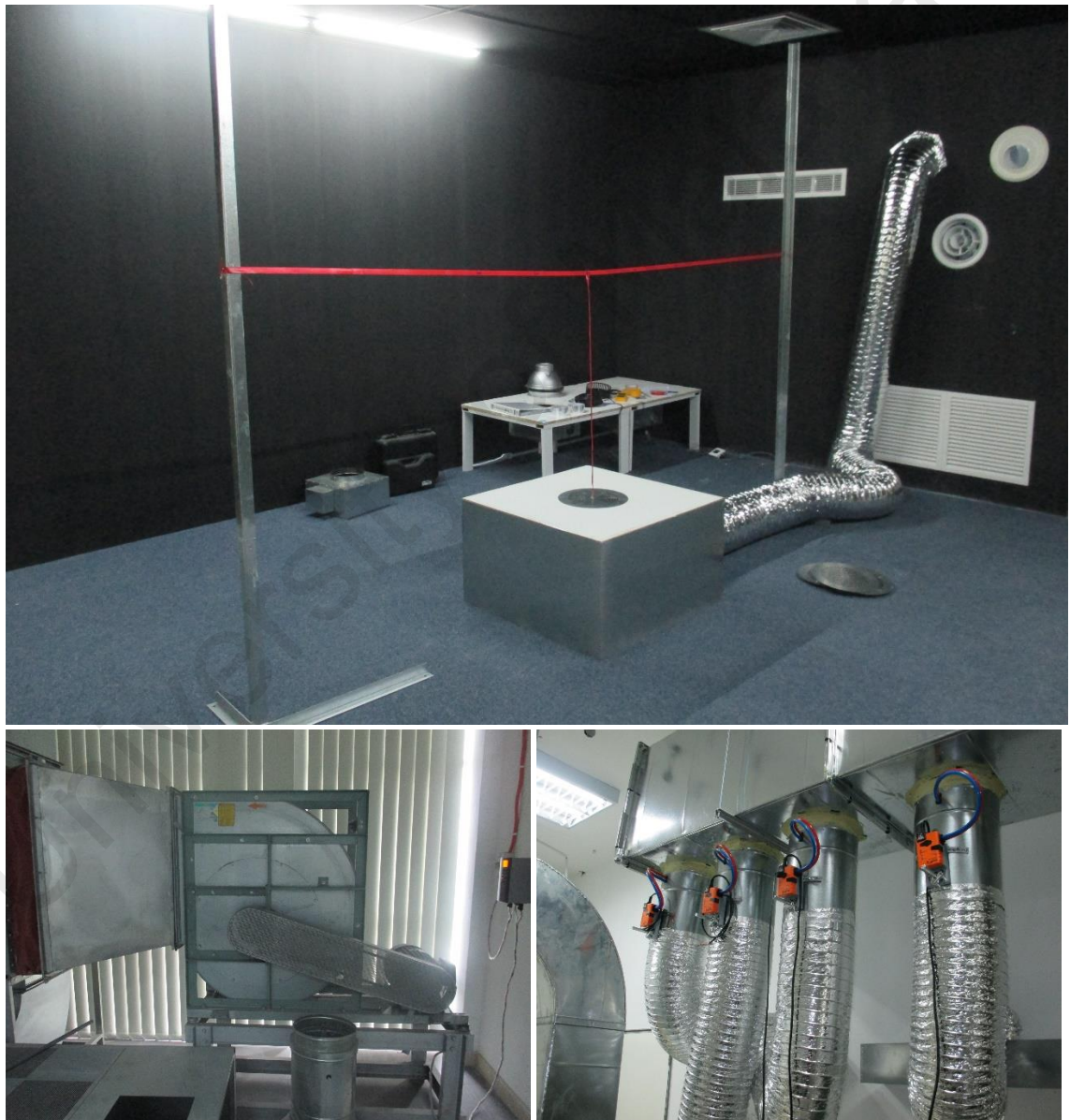
Figure 5.1: Experimental setup for the testing of floor swirl diffuser in laboratory. (Top: floor diffuser installed on the floor plenum with measuring tools, bottom left: supply air VSD fan, bottom right: VAV actuator and damper for airflow rate control).
