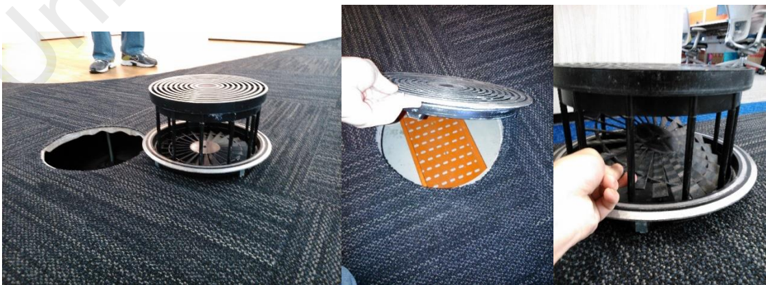
Figure 4.13: Missing, broken and the improper installation of the floor diffuser.
