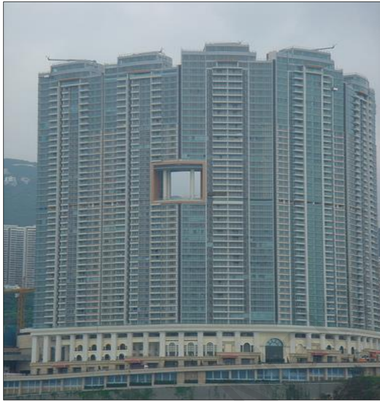
Figure 2.6: A Building In Hong Kong With A Hollow Middle Hole, Engaged Feng Shui Benefits (Lip, 1995)
