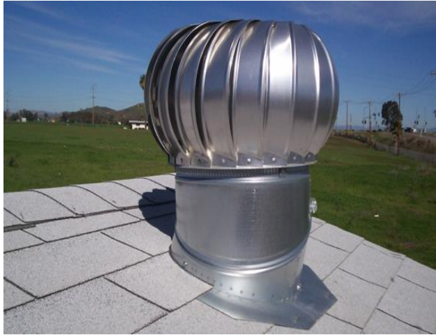
Figure 2.9: Roof turbine (Millette, 2015).
