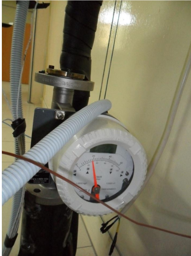
Figure 3. 7: Flow meter settings in the air conditioner unit.
