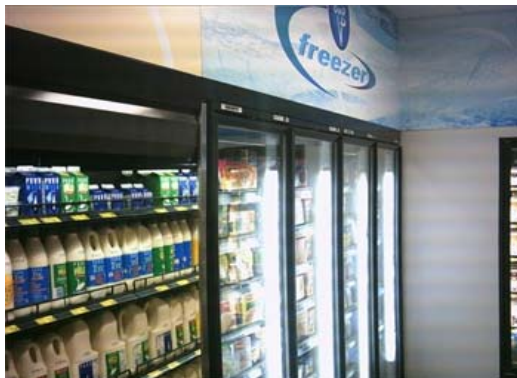
Figure 2.20: Upright chiller used at convenience store
