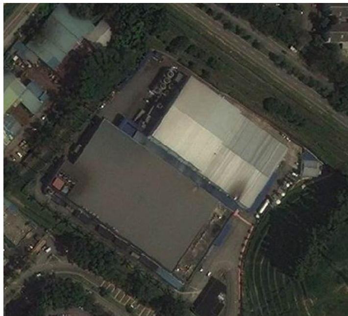
Figure 3.4 Epson Precision building satellite view
