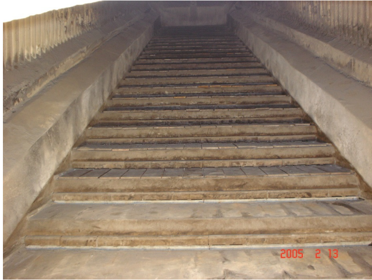
Figure 5.2: Reciprocating grate internal view
