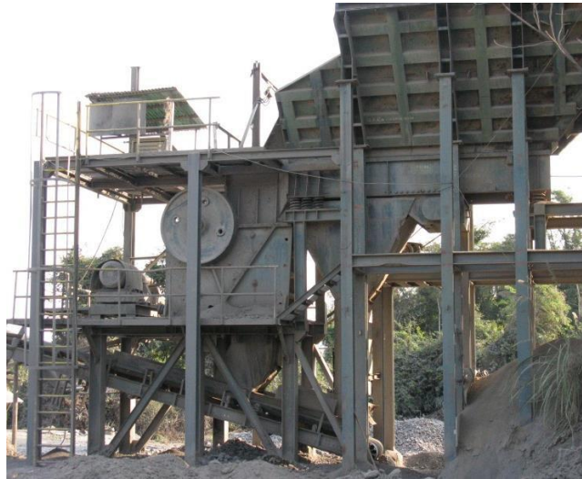
Figure 3.3 Primary crushed stage
