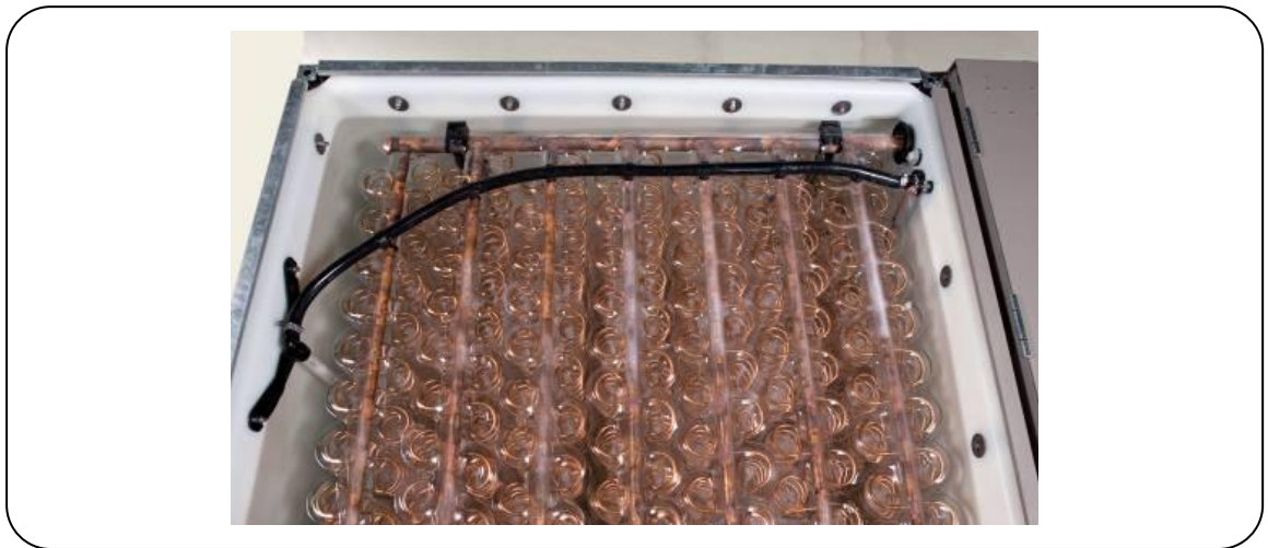
Figure 2.8: A photograph of an external melt ice-on-coil system (sub-systems of an Ice-Bear® unit) (ice-energy).
