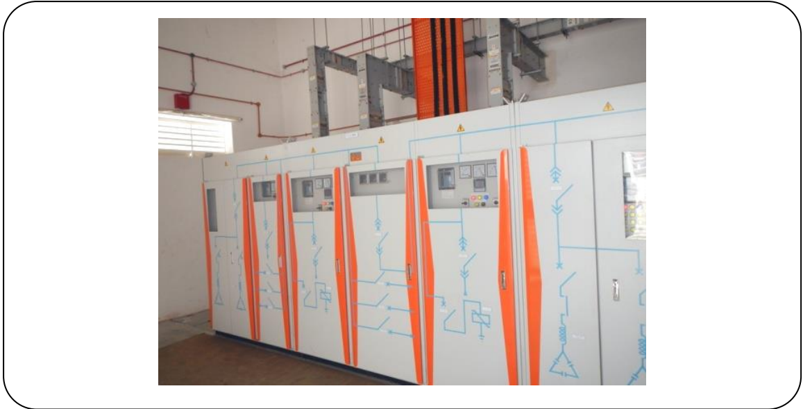
Figure 3.5: The main distribution cabinet.
