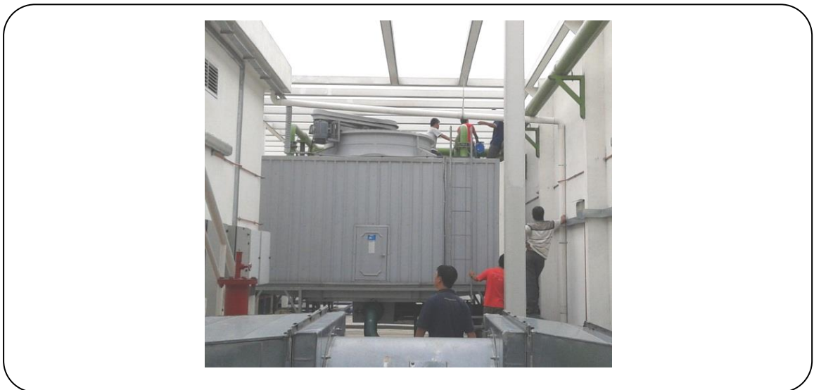
Figure 3.9: Cooling tower, during maintenance.
