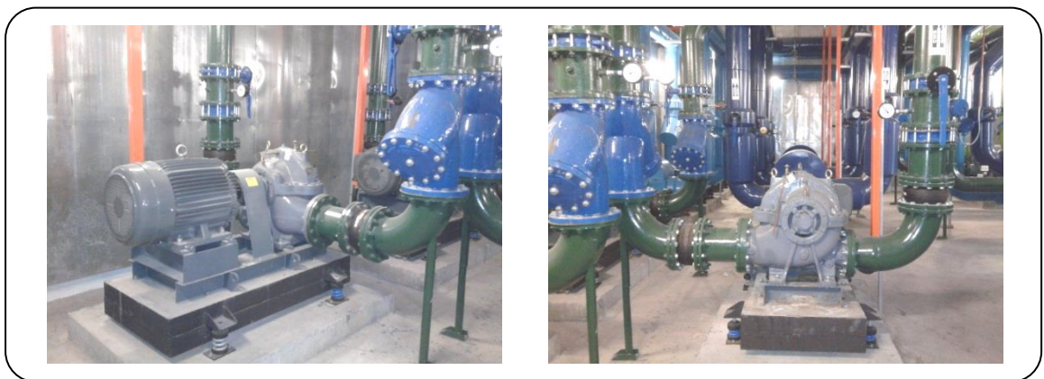
Figure 3.8: Horizontal split casing pump.
