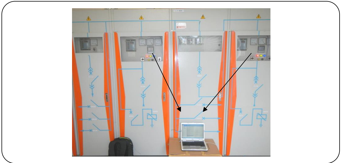
Figure 3.16: The power monitoring system setup inside the electrical room. The computer is logging the data from two PAC3200 power analysers.
