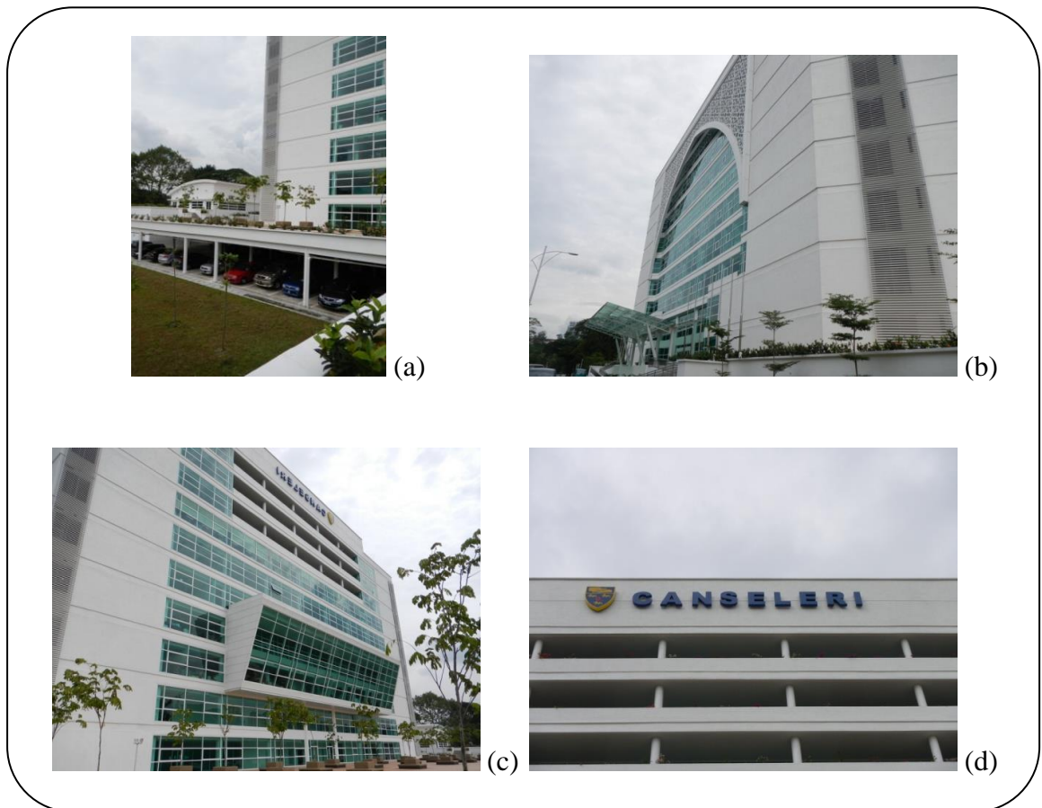
Figure 3.4: (a) Northern face, (b) Southern face and (c) the underground of the building.
