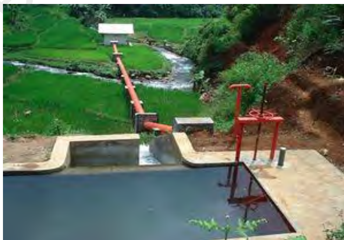
Figure 2.7: Run-of-River hydropower plant (Energylopedia, 2016)
