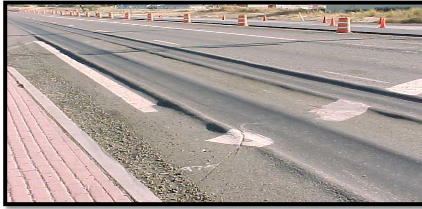
Figure 2.6: Rutting (source: Pavement Interactive, 2008)
