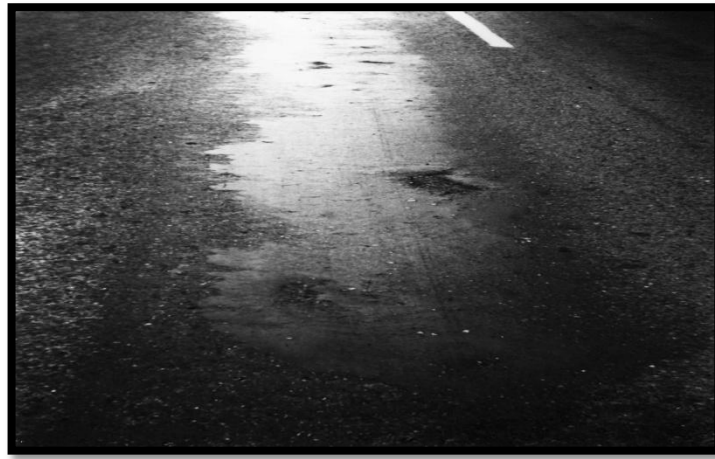
Figure 2.9: Bleeding (source: Asphalt Institute, 2009)
