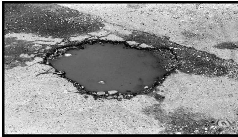
Figure 2.8: Potholes (source: Asphalt Institute, 2009)
