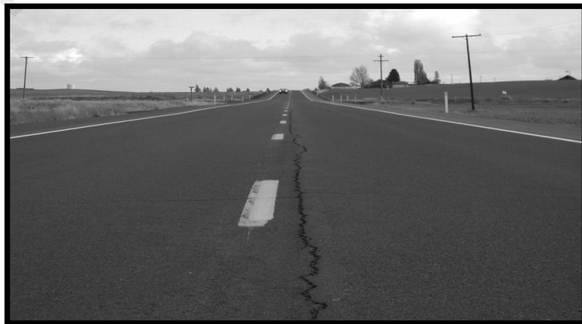
Figure 2.4: Longitudinal cracking (source: Asphalt Institute, 2009)
