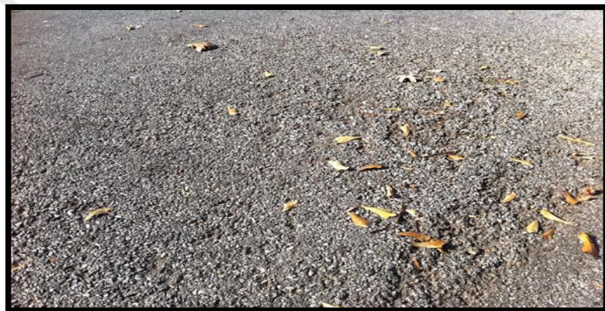
Figure 2.7: Ravelling (source: Neal, 2007)
