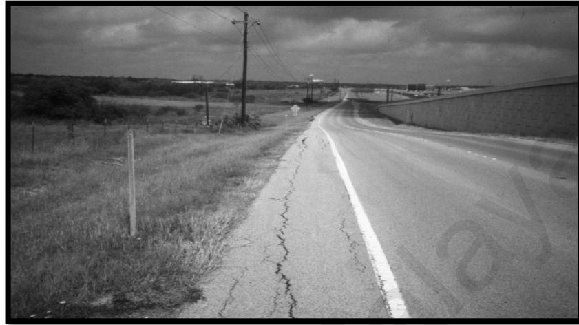
Figure 2.2: Edge Cracking (source: Asphalt Institute, 2009)
