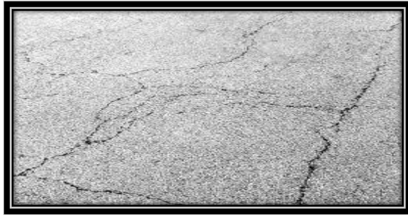
Figure 2.3: Block Cracking (source: Asphalt Institute, 2009)
