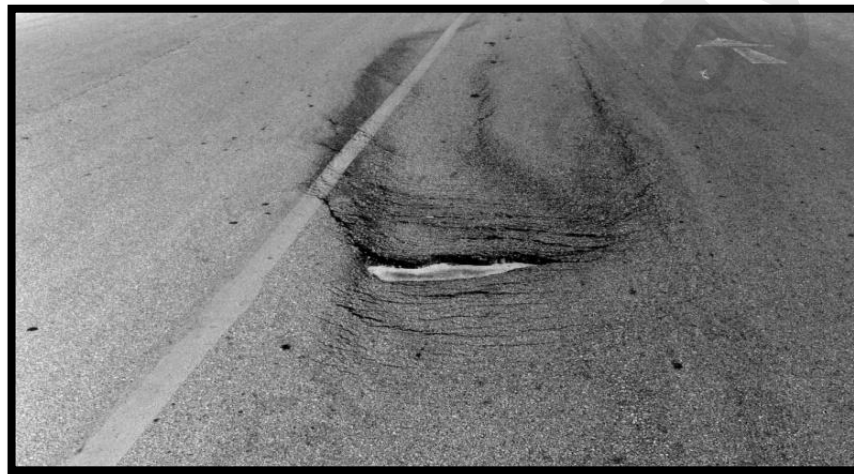
Figure 2.5: Slippage cracking (source: Asphalt Institute, 2009)
