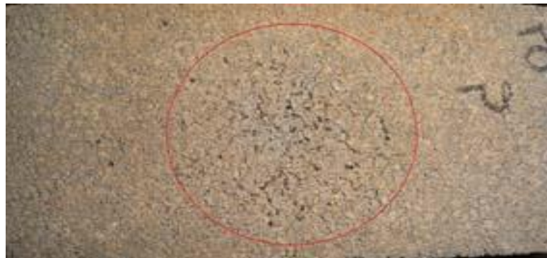
Figure 4.16: Appearance of the eroded bricks
