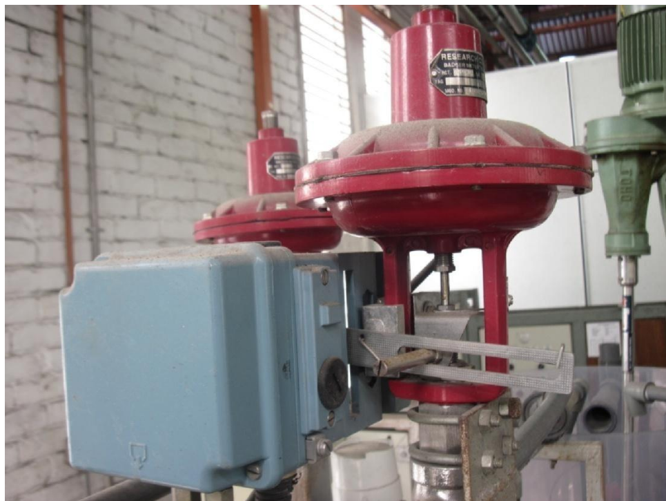
Figure 5.5: Control valves (acid and base) used in the pilot plant
