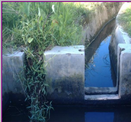
Figure 3.7 Debit, sediment, clogged rubbish and overgrown problems at site study Pante Lhong technical irrigation system
