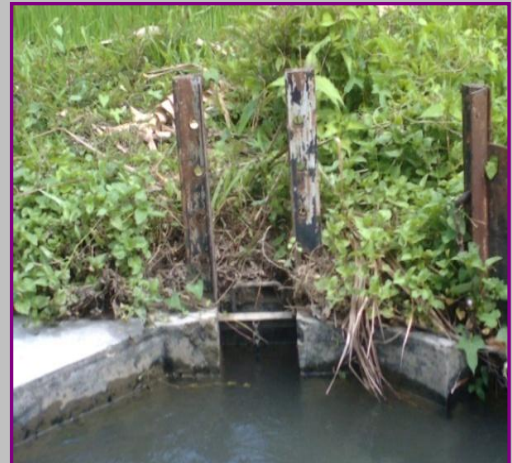
Figure 3.7 Debit, sediment, clogged rubbish and overgrown problems at site study Pante Lhong technical irrigation system
