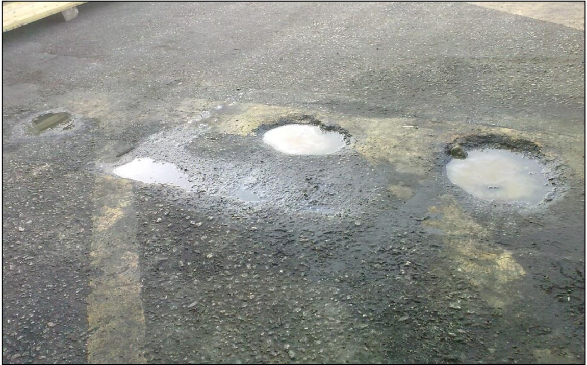
Figure 5.8 Potholes spotted at forklift route
