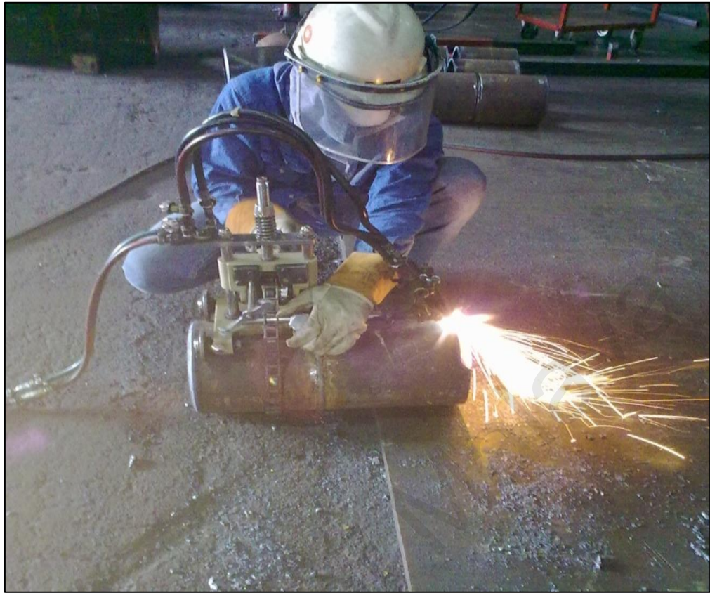
Figure 5.5 A pipe fitter cutting a pipe coupon using oxy-acetylene gas cutter
