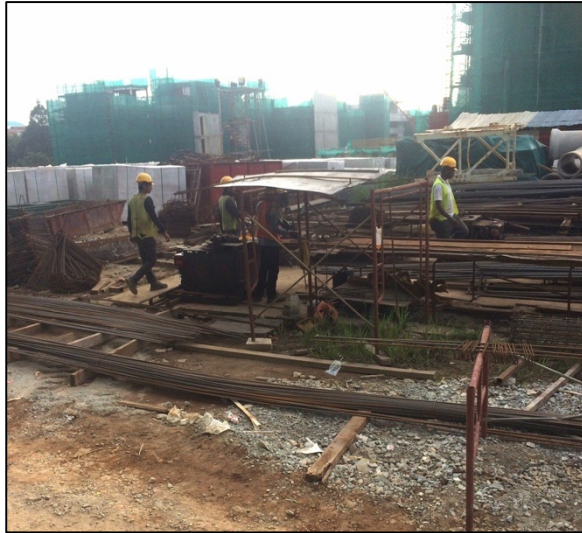
Figures 4.1 Bar bending machine in the bar bending yard
