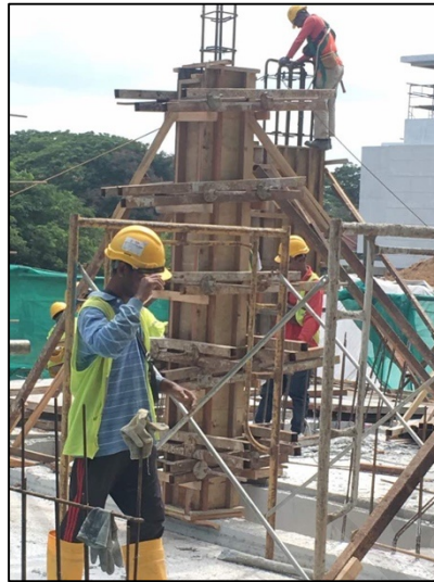
Figures 3.2 Photo of workers customizing the timber formwork
