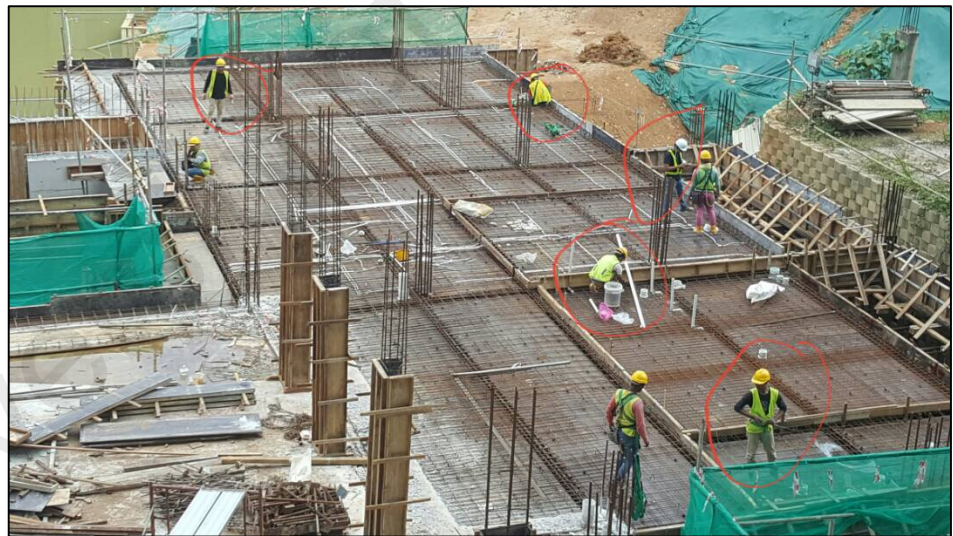
Figures 3.3 Photo of electrical worker laying the pipe
